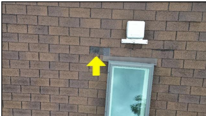
2. Missing, loose or torn
