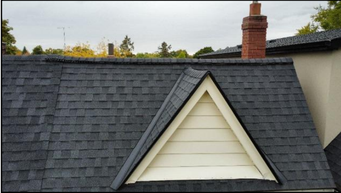
1. Asphalt shingles -- Good condition
