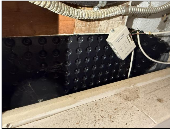
27. Interior drainage system example
