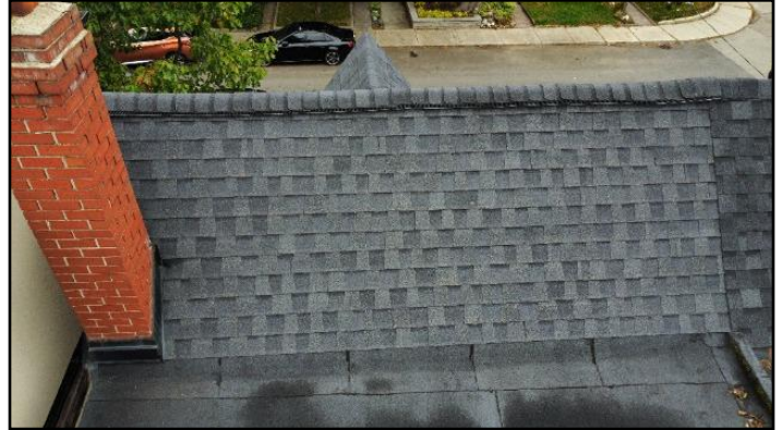
2. Asphalt shingles -- Good condition
