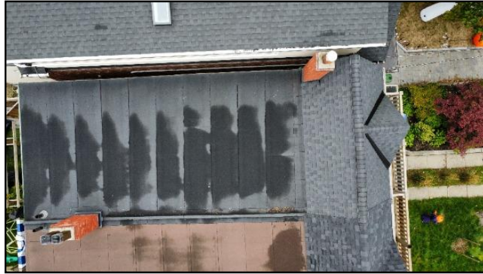
6. Full roof view from drone
