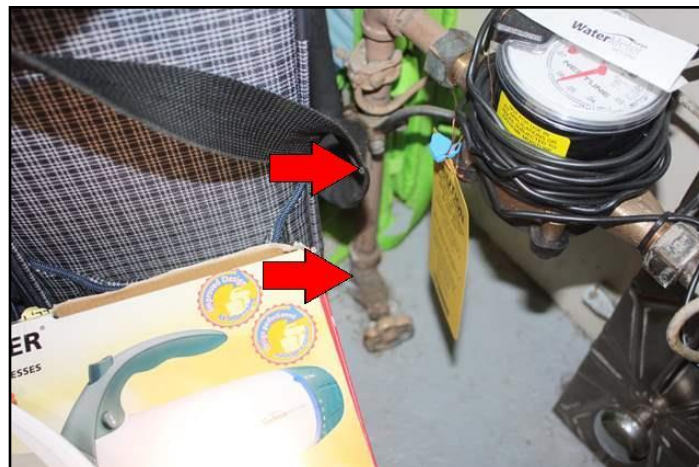
Galvanized steel supply pipe should be...
