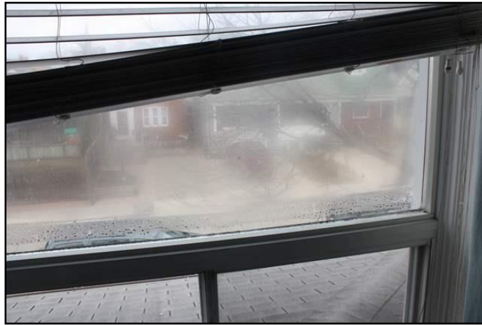
Lost seal on double or triple glazing
