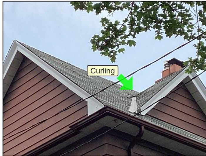
Curling, deteriorating shingles
