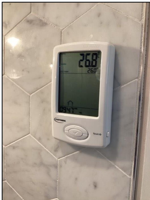
Upstairs floor heat controls
