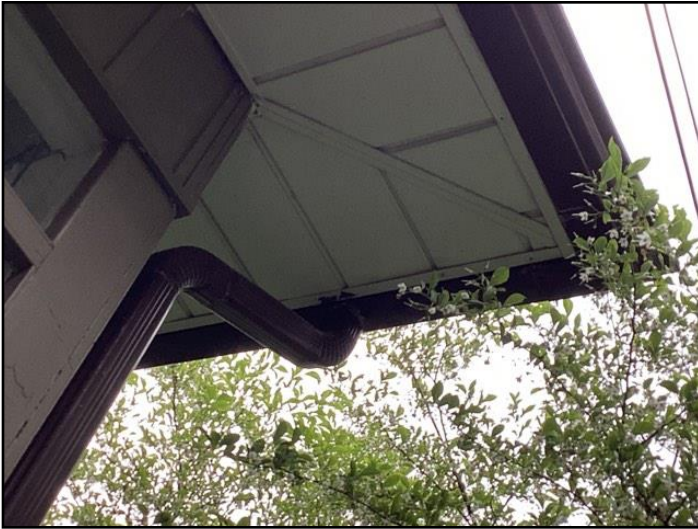
Gutter and downspout
