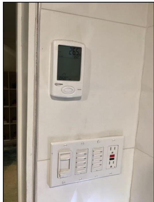
Basement floor heat controls
