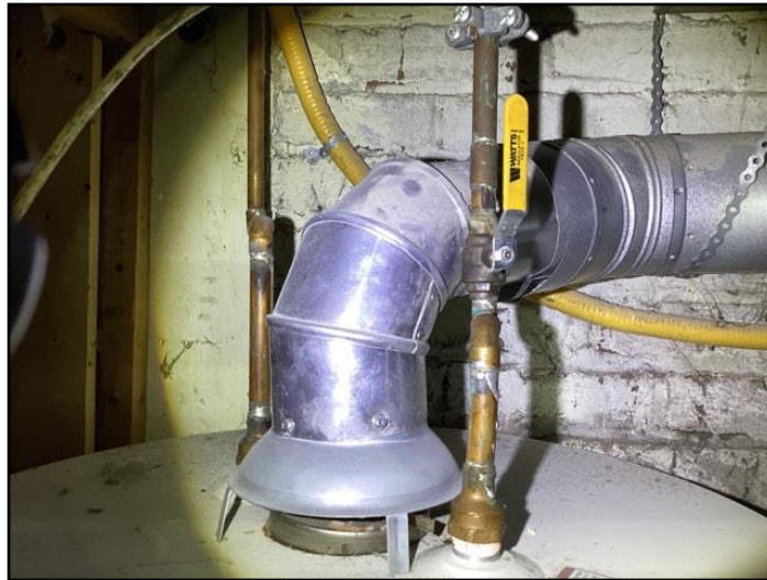
Water Heater direct vent and water shut-off
