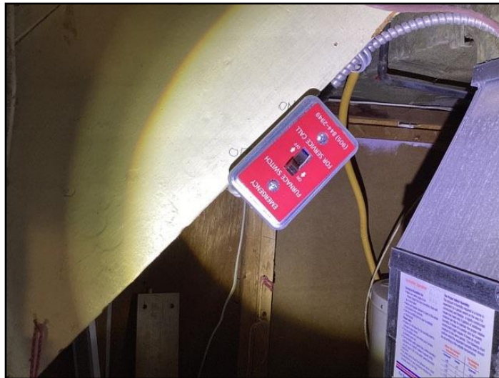
Furnace shut-off
