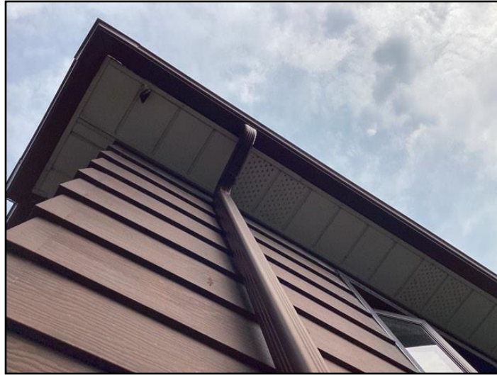
Soffit with vents
