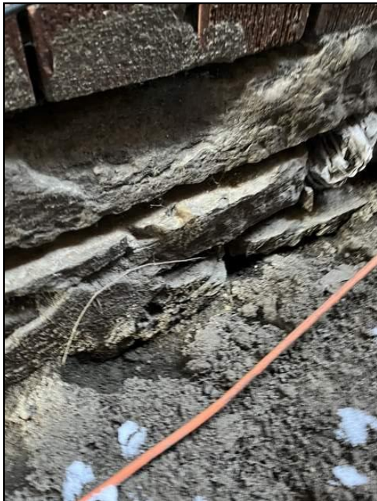
18. Mortar deteriorated or missing
