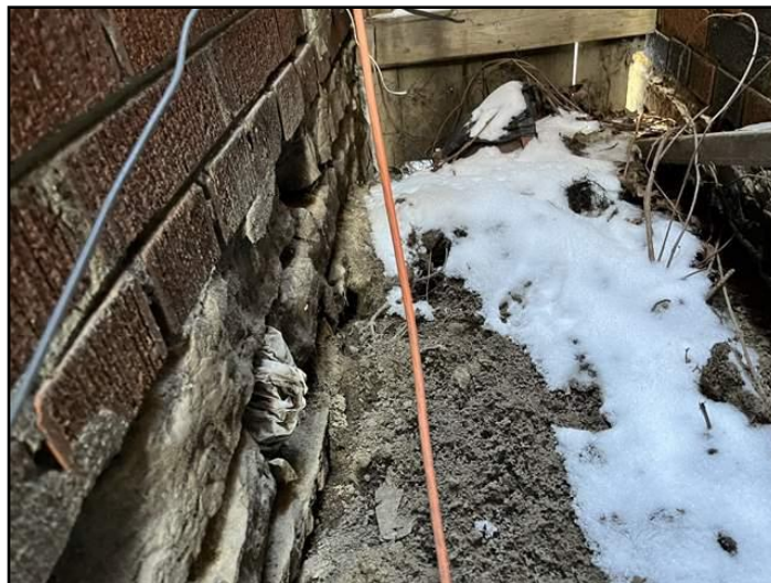
22. Parging damaged or missing
