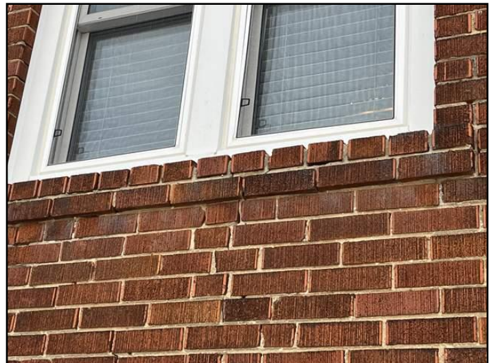
9. Mortar deterioration
