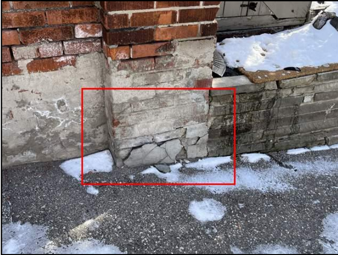
20. Parging damaged or missing
