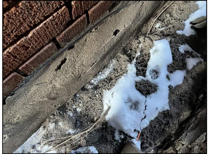
21. Parging damaged or missing
