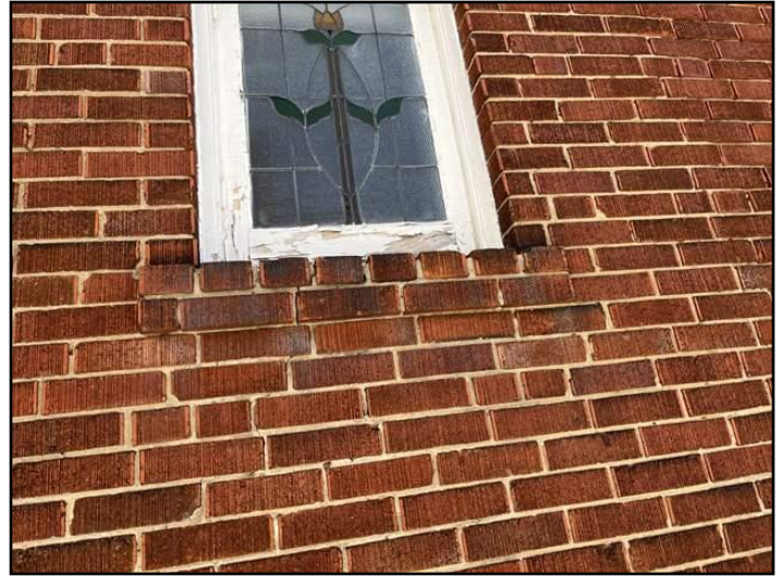
11. Mortar deterioration
