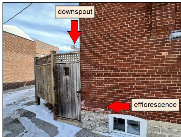
6. Should discharge 6 feet from building
