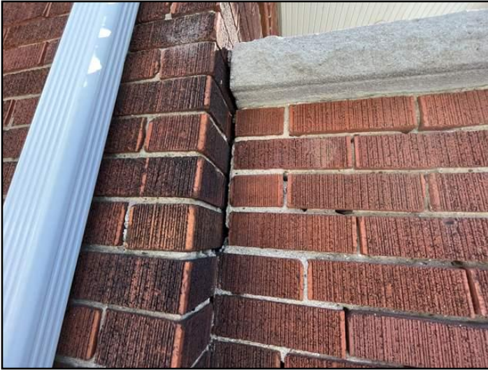
10. Mortar deterioration
