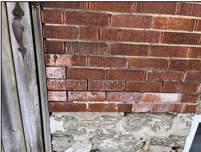
8. Mortar deterioration
