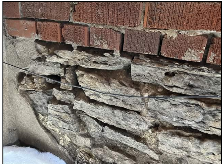
19. Mortar deteriorated or missing
