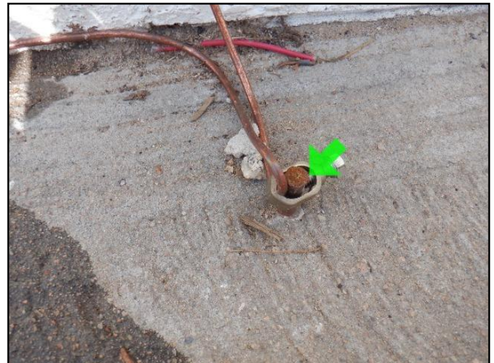
49. Copper - water pipe and ground rod
