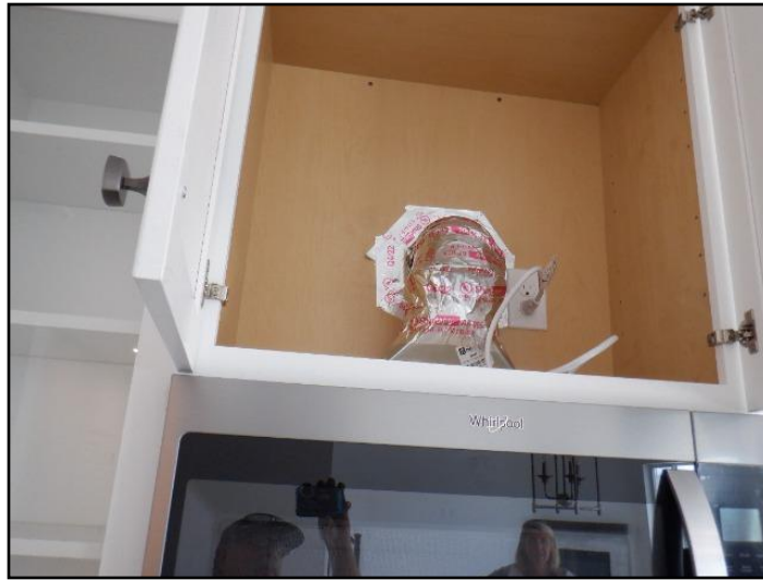
110. Exhaust fan discharges to the exterior
