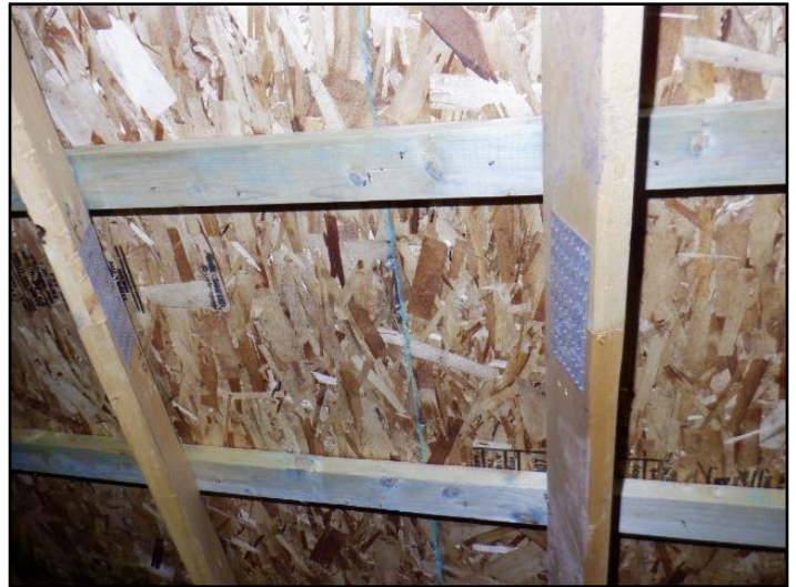
39. Engineered Trusses appeared to be in good...
