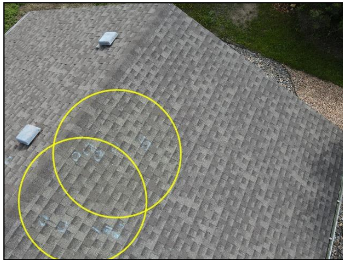
19. Evidence Of Hail Damage
