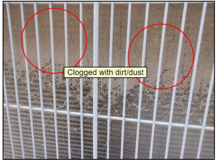
71. Dust/Debris in cooling fins, reduced...
