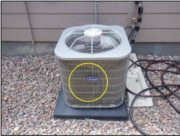
70. Dust/Debris in cooling fins, reduced...
