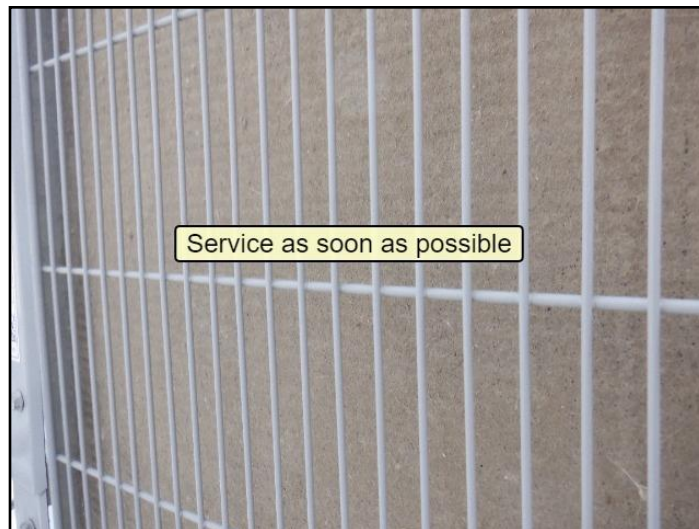
72. Dust/Debris in cooling fins, reduced...
