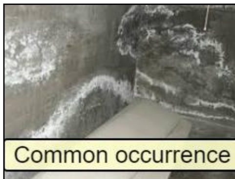
100. Efflorescence
