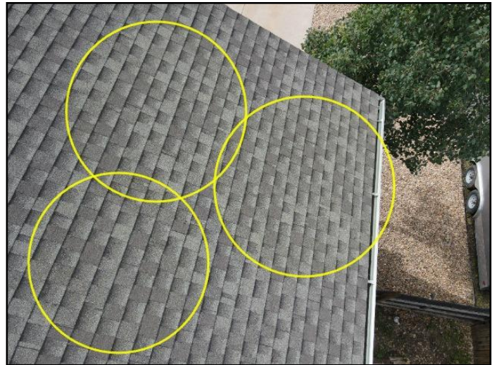
18. Evidence Of Hail Damage
