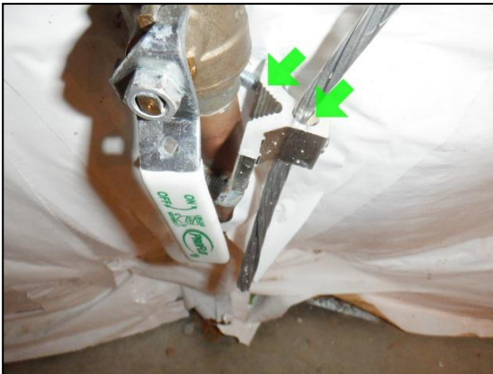
48. Copper - water pipe and ground rod
