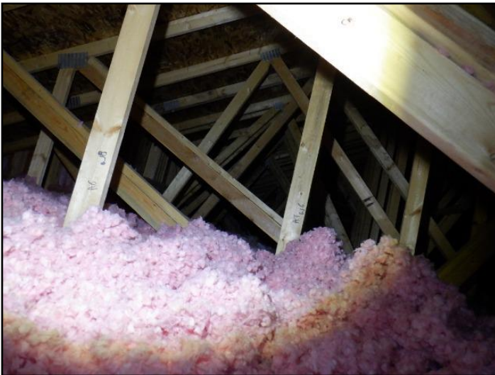
40. Engineered Trusses appeared to be in good...
