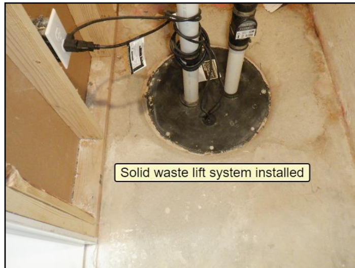
89. Solid waste pump (ejector pump)
