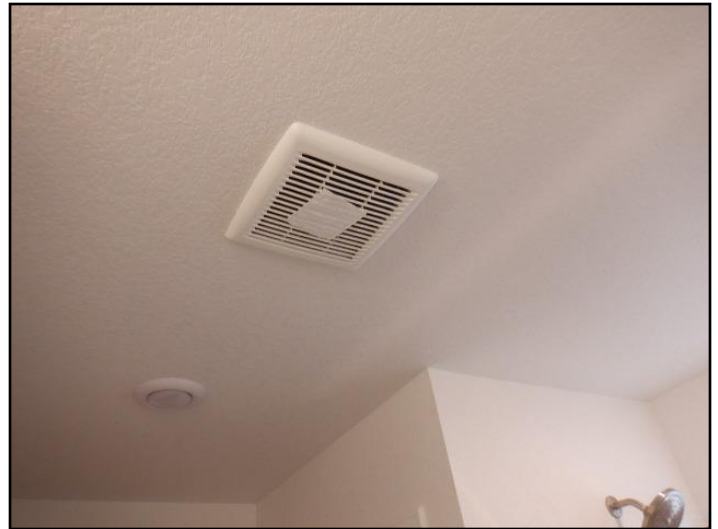
112. Bathroom fan(s) operated and have good air...
