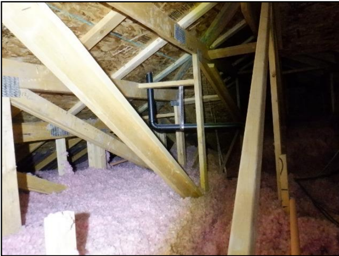
38. Engineered Trusses appeared to be in good...
