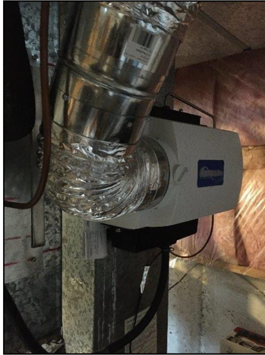
20. Duct mounted bypass humidifer
