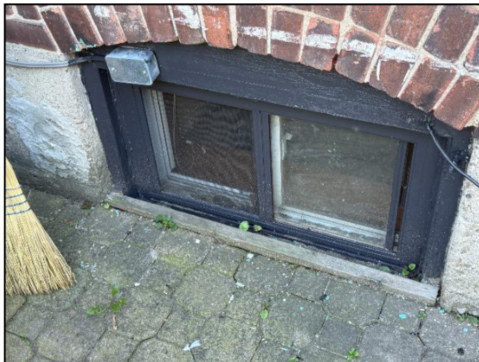
12. Sill - Near or at Grade Level
