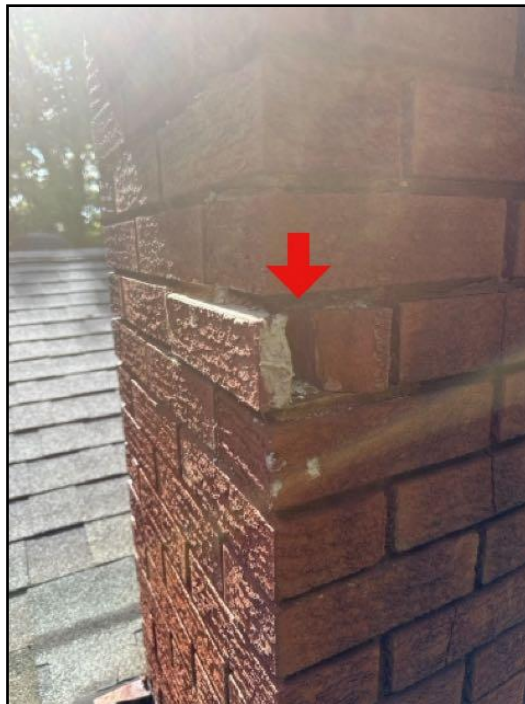
118. Spalling
