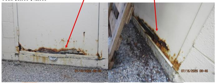
Seals are warped/loose damaged on various windows and at glass doors. Some transition flashing is poor and there is evidence of water intrusion around the bottom of the door at various entrances. Window/door seal repairs are needed in various areas at approximately 16 windows/doors.
