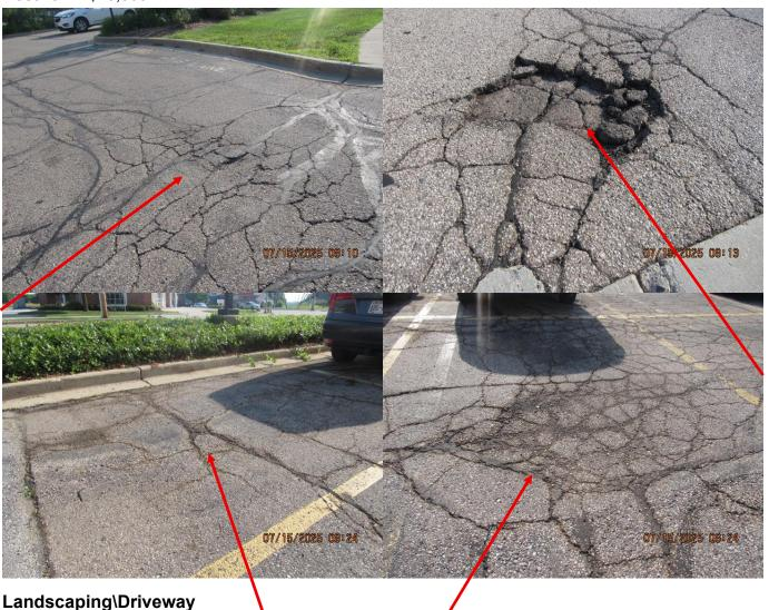
13. Approximately 190,000 square feet of parking lot is in need of repairs including patching, sealing and new painted lines.
