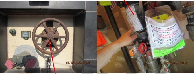
44. There appears to be old/abandoned fire sprinkler system components that are rusted out. It appears that these components are not being used.
