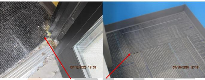
53. The carpet is loose and should be secured. This could also potentially become a trip hazard.
