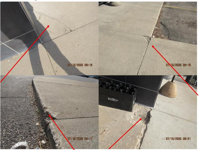
12. The concrete walkways have damage in various areas. Some areas are deteriorated. Some areas are cracked. Curbing is also damaged in various areas. A Concrete contractor should be consulted to evaluate the concrete walkways/curbing throughout for repairs.
