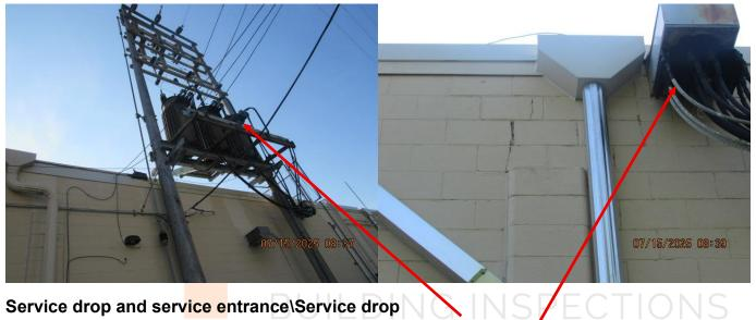
20. Transformers show signs of rusting. Birds nests were noted at the transformers and service drops, fencing is rusted and damaged on the roof. WE energies and/or A commercial Electrician should be consulted for improvements in this area.
