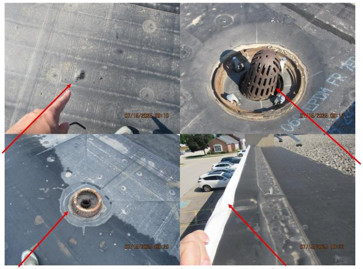
Roof repairs are needed in the newer rubber roof systems on the buildings. Some drains and drain covers are poor. Some seams are poor in the smaller building and damage was noted in the smaller building roof system. A Certified Roofer should evaluate the roof systems for repairs.
