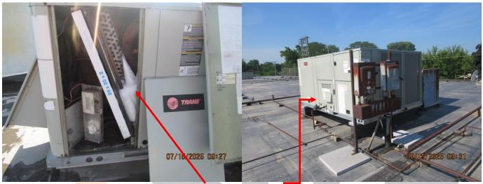
34. The Roof top units on the main building and heating systems in the small building are in need of service/maintenance. Some units show signs of corrosion, rust, neglect, poor function. A Commercial HVAC contractor should be consulted.
