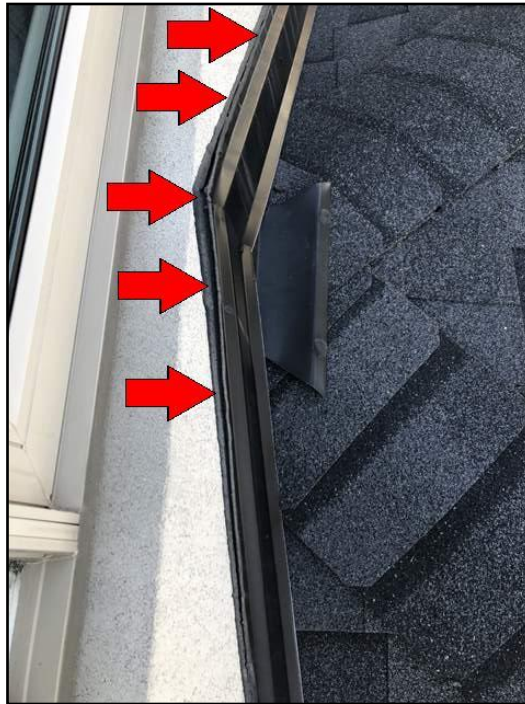
2. Damage, loose, open seams, patched
