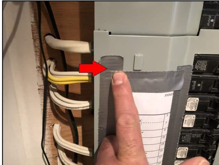
20. Missing or Improper Panel Cover Fasteners
