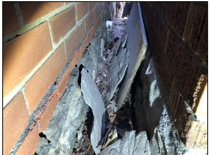
13. Parging damaged or missing
