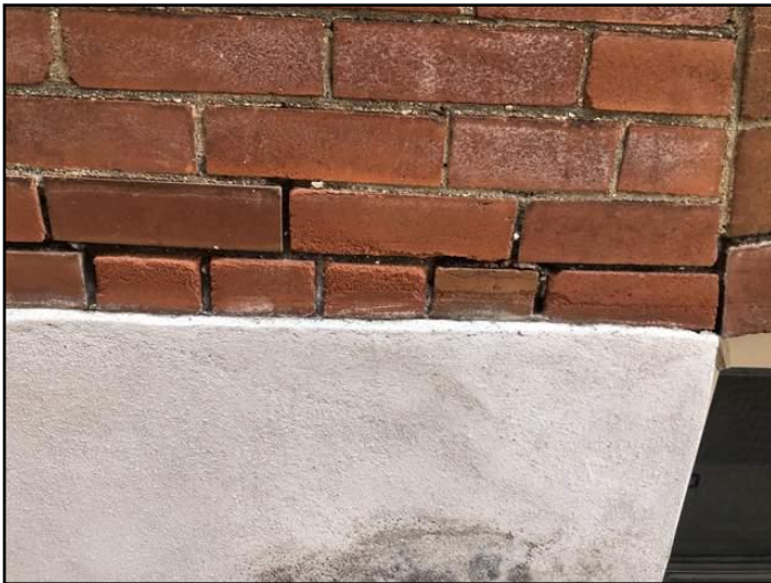
15. Mortar deteriorating
