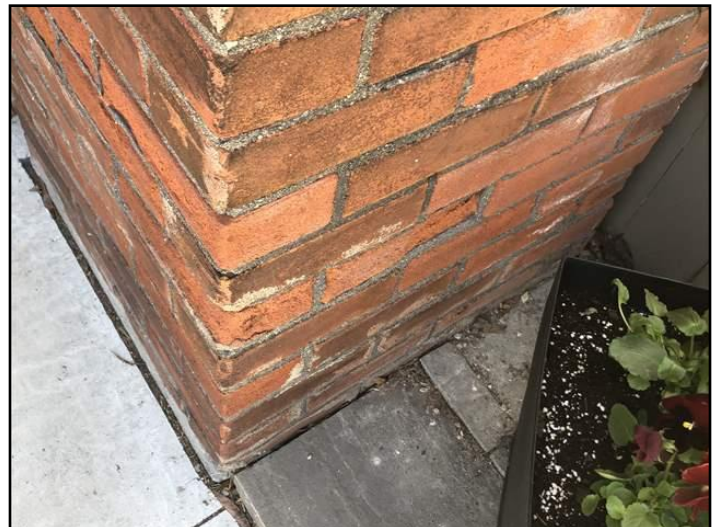
6. Spalling
