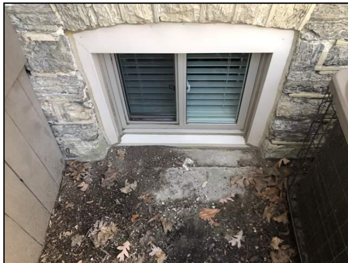
8. Sill - Near or at Grade Level
