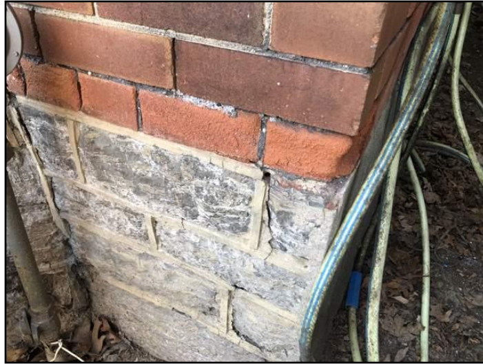
7. Spalling
