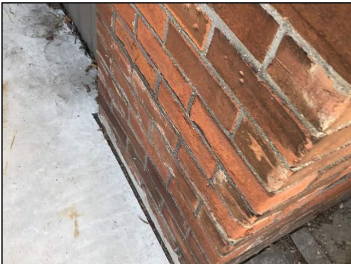
5. Spalling
