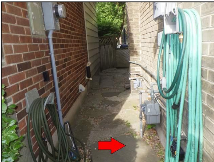
Improper slope or drainage
