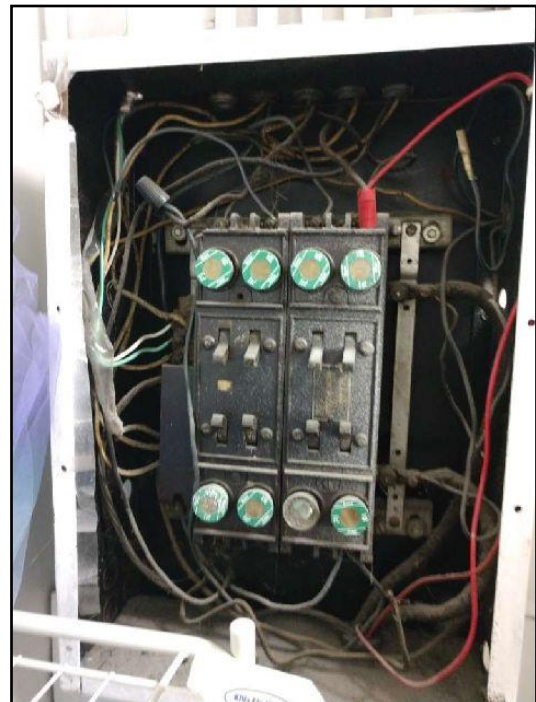
49. Abandoned wires in panel
