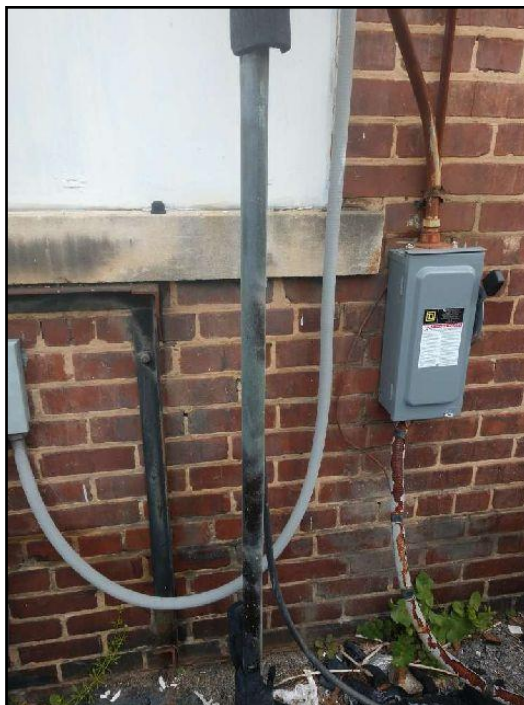
60. Insulation - missing
