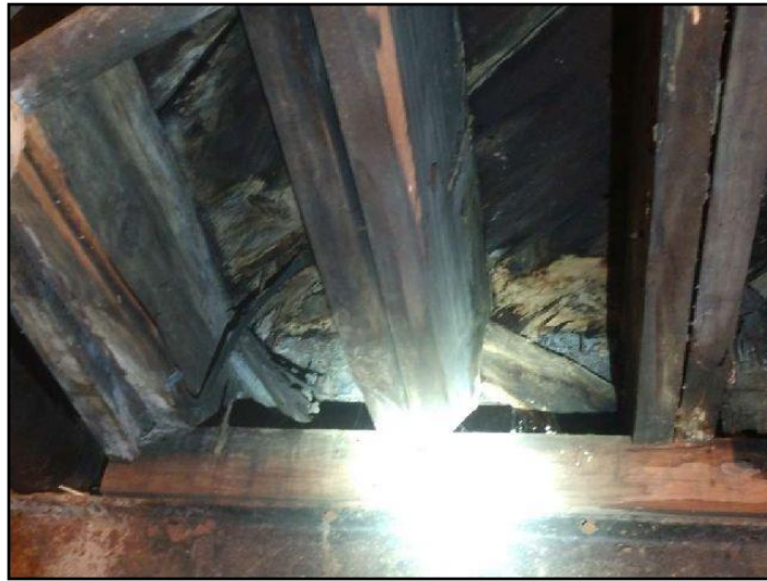
125. Rot or insect damage
