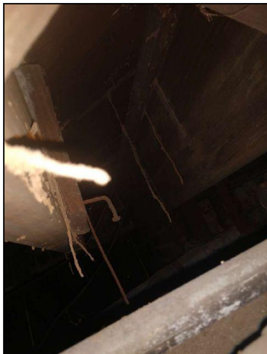
27. Suspected Fungal growth on framing. Organic...
