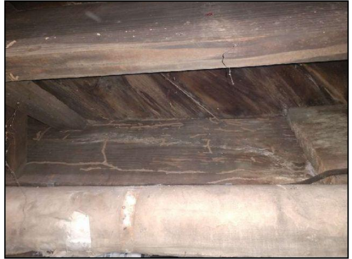
37. Rot, insect or fire damage
