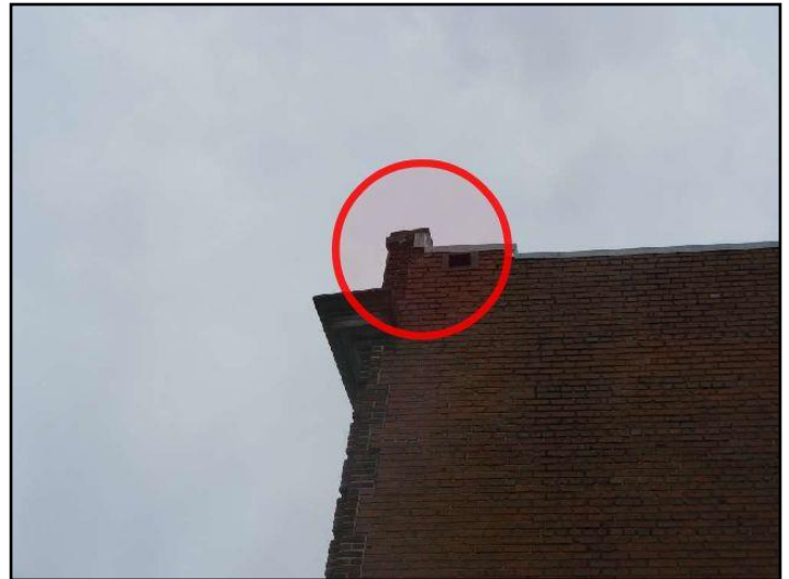
93. Masonry deterioration
