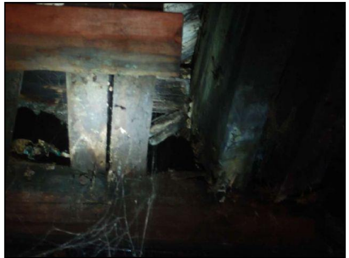
124. Rot or insect damage
