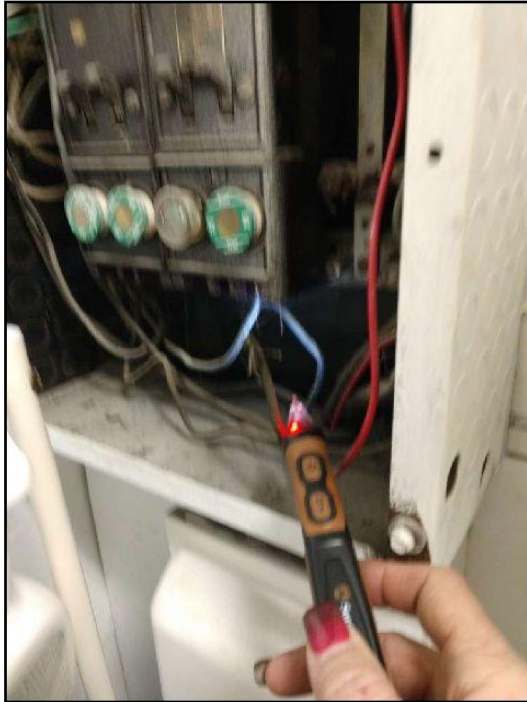
138. Abandoned wires in panel
