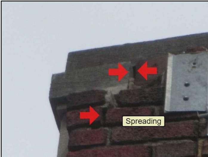
4. Masonry deterioration
