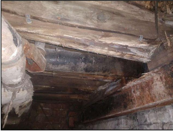
126. Rot, insect or fire damage
