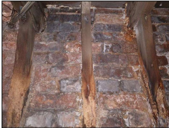
135. Masonry walls are weeping
