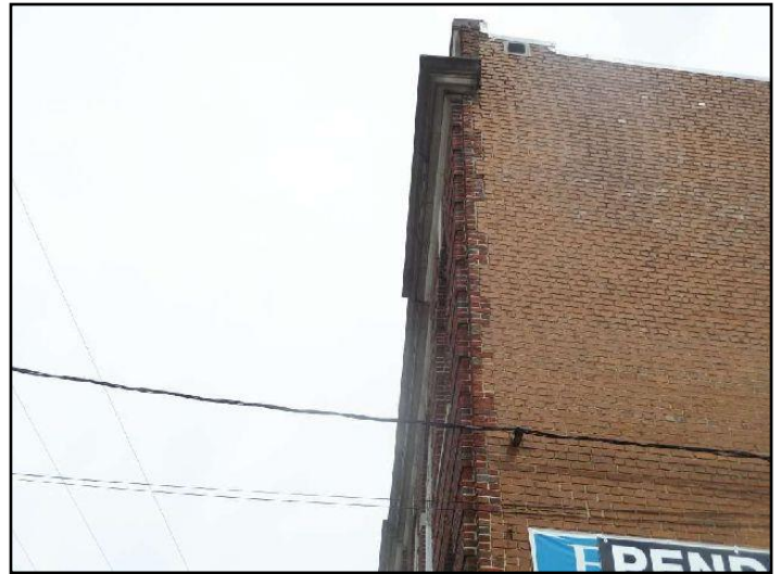
95. Masonry deterioration
