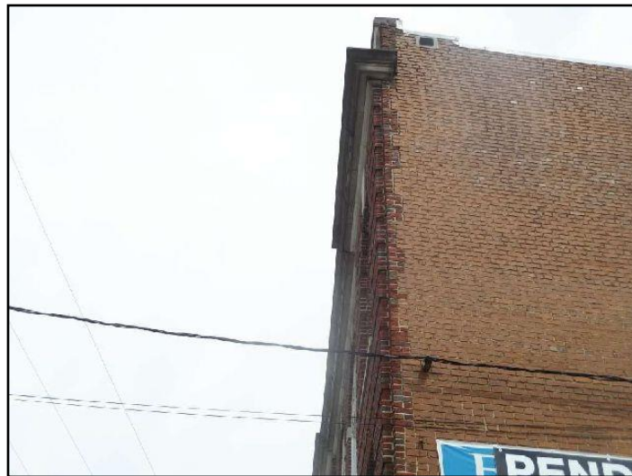
7. Masonry deterioration
