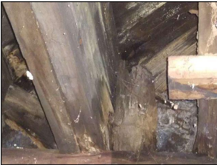
123. Rot or insect damage
