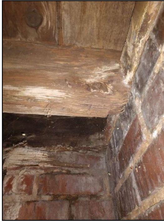
129. Rot, insect or fire damage
