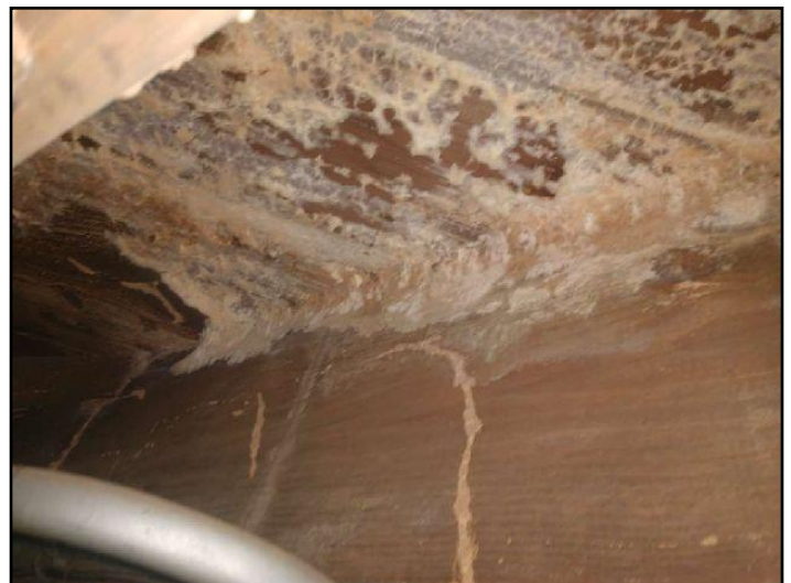
28. Suspected Fungal growth on framing. Organic...
