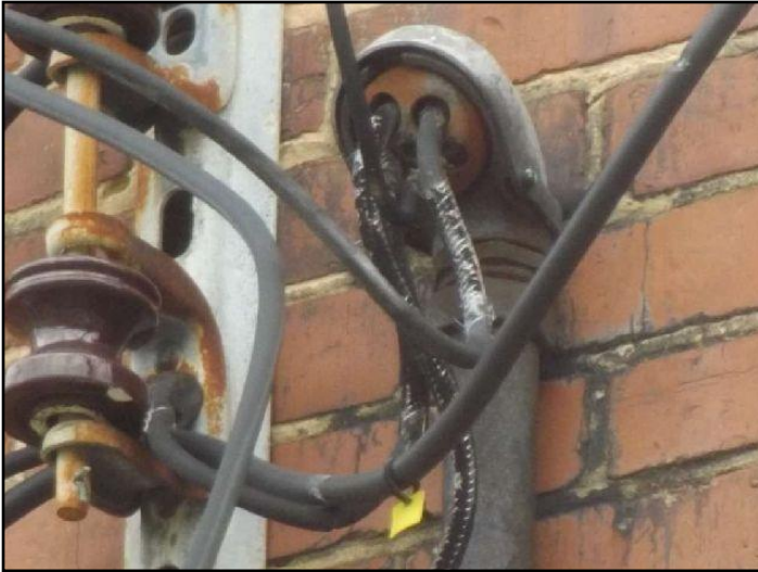
46. Insulation missing or damaged
