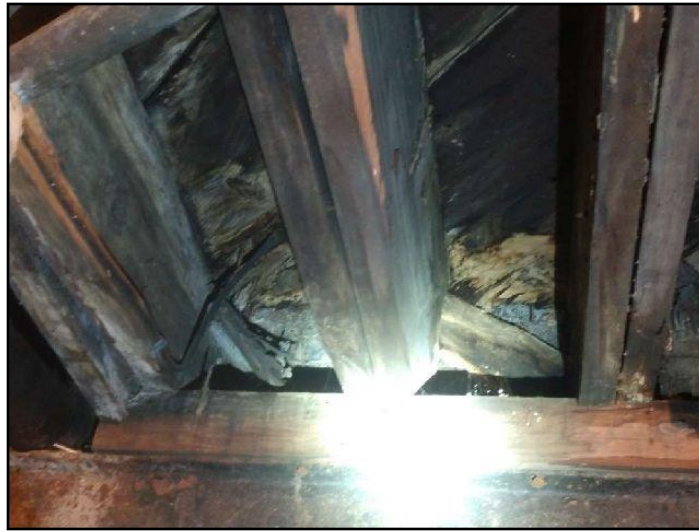
35. Rot or insect damage
