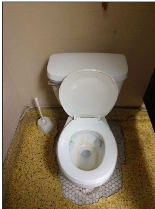
182. Toilet loose at floor - Note: This inspecto...
