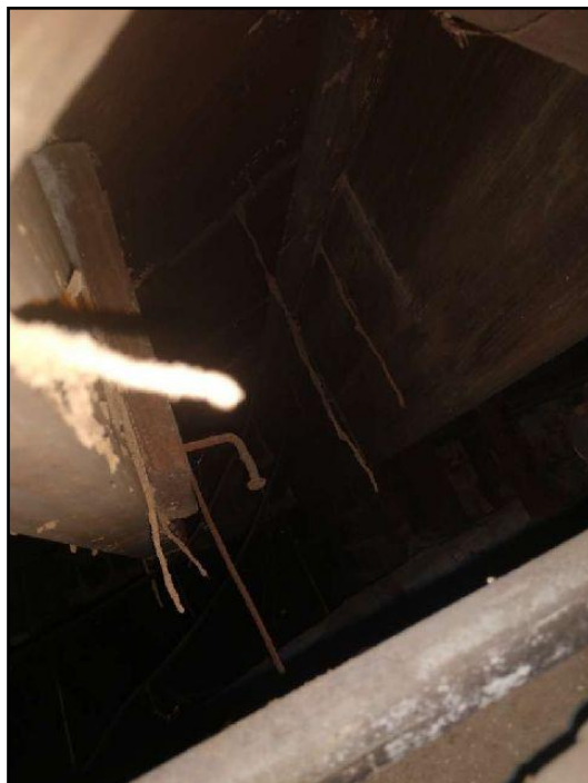
117. Suspected Fungal growth on framing. Organic...
