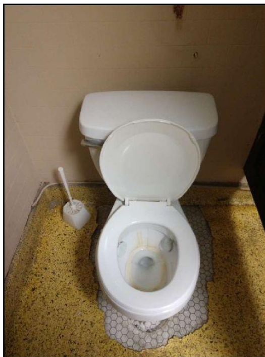
67. Toilet loose at floor - Note: This inspecto...
