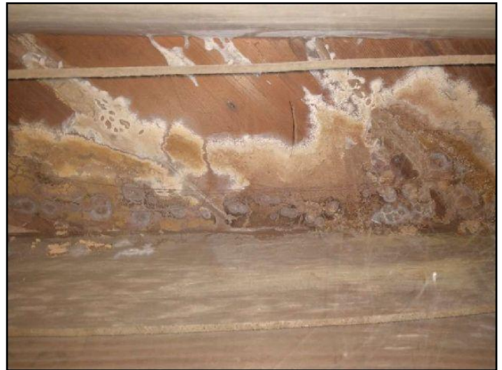
24. Suspected Fungal growth on framing. Organic...
