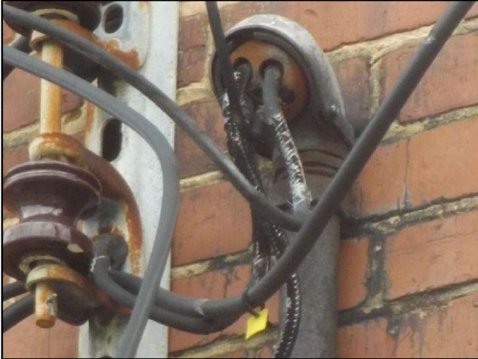
136. Insulation missing or damaged
