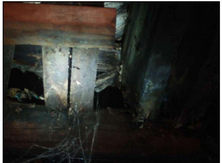
34. Rot or insect damage
