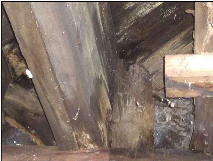
33. Rot or insect damage
