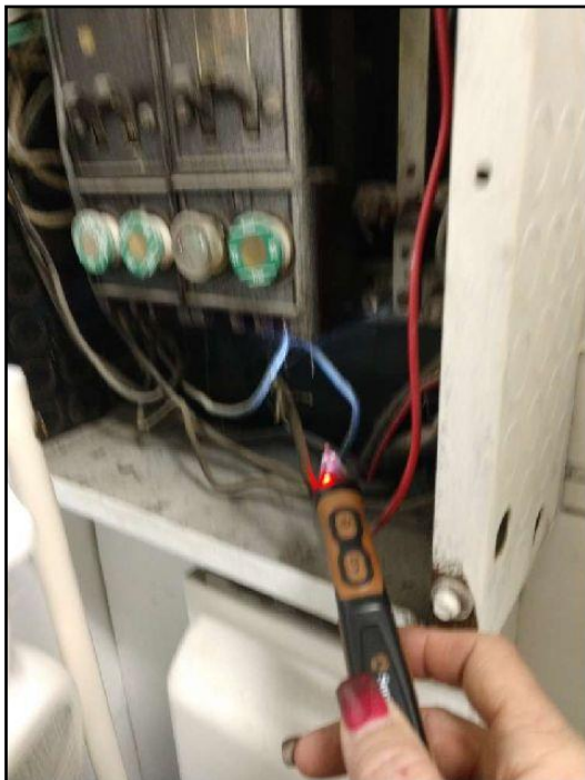
48. Abandoned wires in panel
