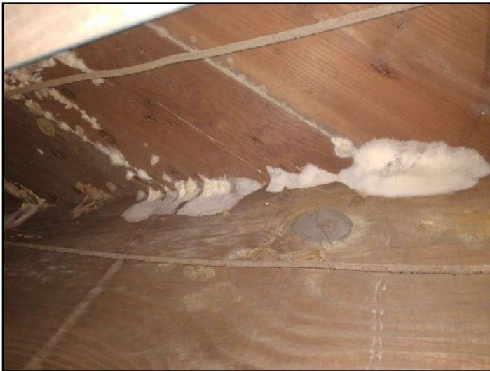
113. Suspected Fungal growth on framing. Organic...
