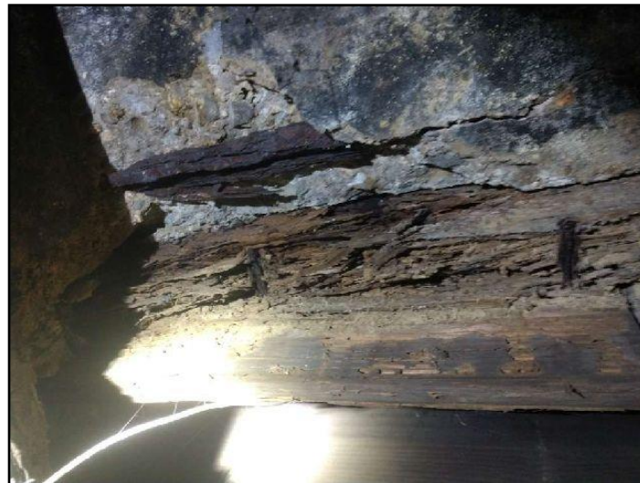
130. Rot, insect or fire damage
