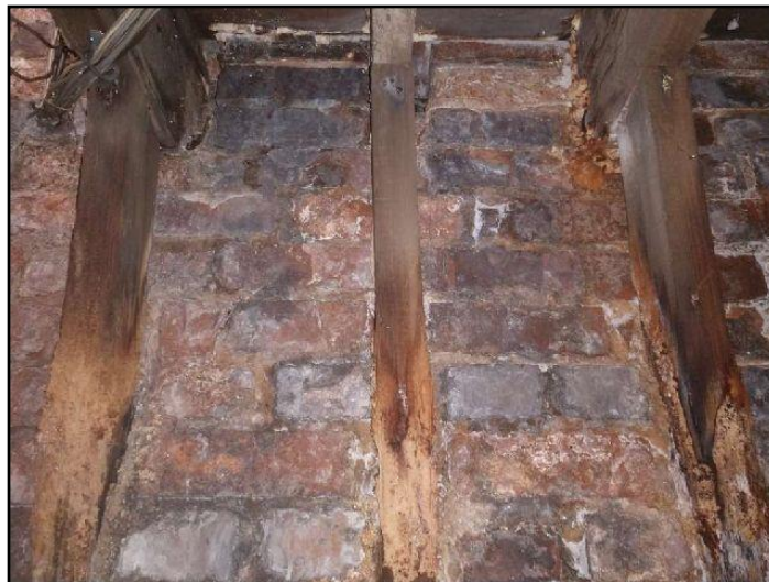
45. Masonry walls are weeping
