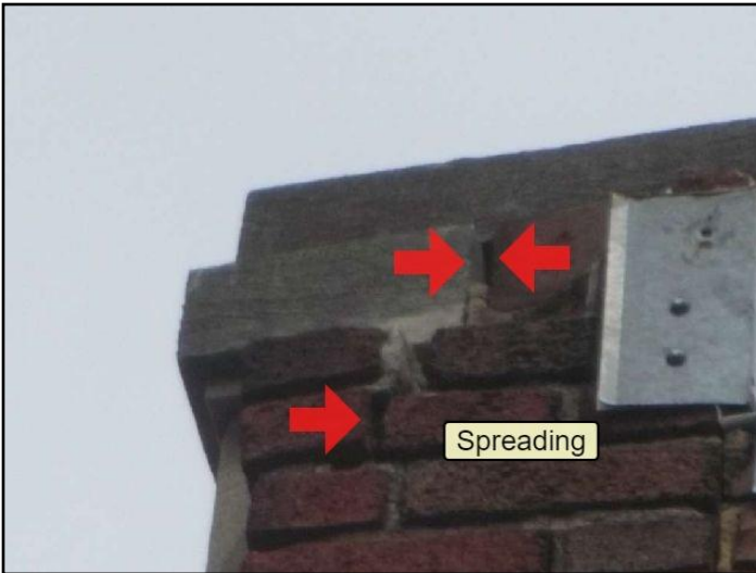
92. Masonry deterioration
