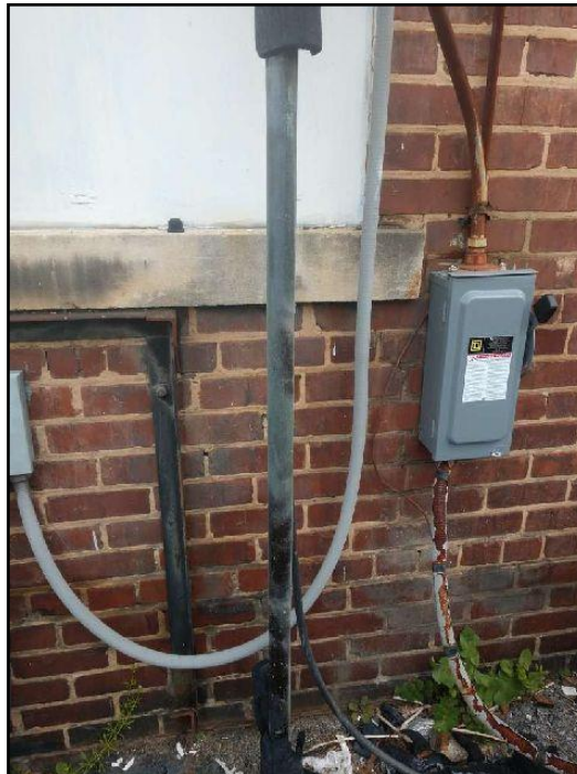
159. Insulation - missing
