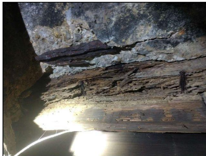
40. Rot, insect or fire damage
