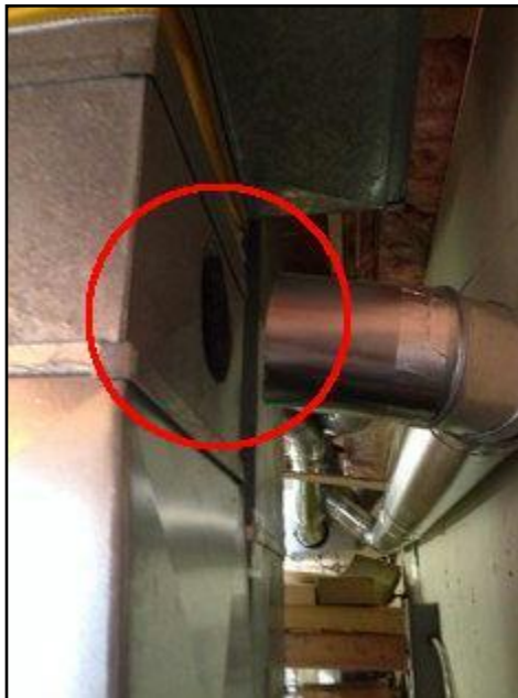
Warm-side fresh air duct not well-connected t
