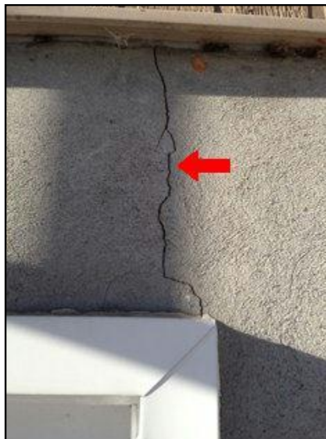
Minor Cracks
