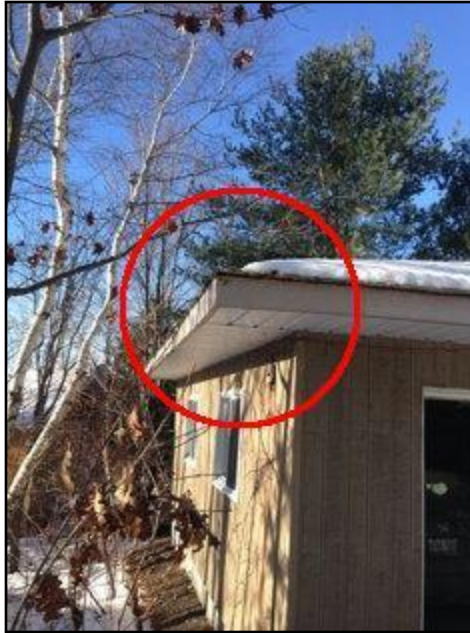
Gutters Missing
