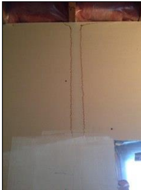
Minor water damage
