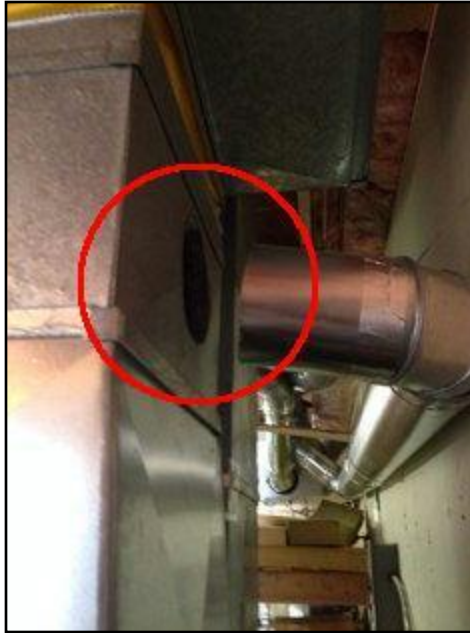
Warm-side fresh air duct not well-connected t
