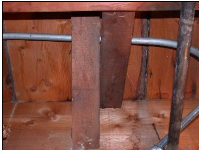
5. Note bridging used properly where seen
