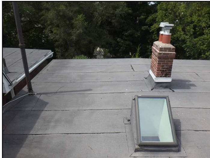
Modified bitumen membrane
