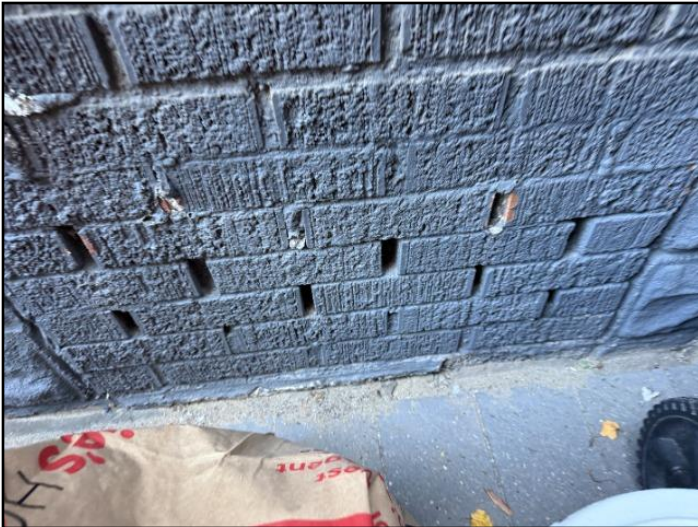
10. example of mortar deterioration
