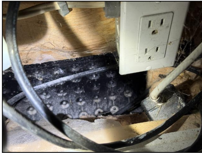
27. Drainage membrane at interior
