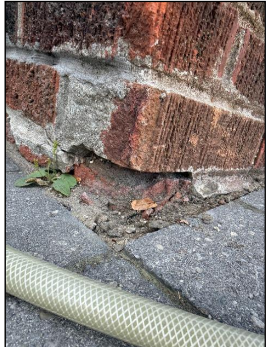
11. example of spalling at column
