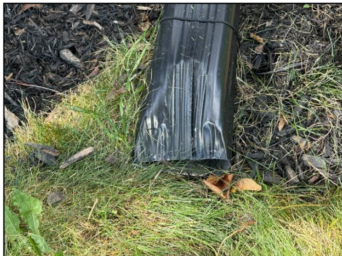
13. Minor damage at downspout
