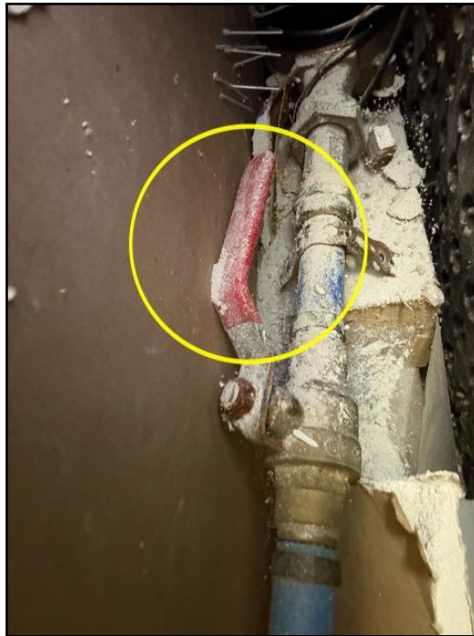
26. Main water shut off valve - Front of the...
