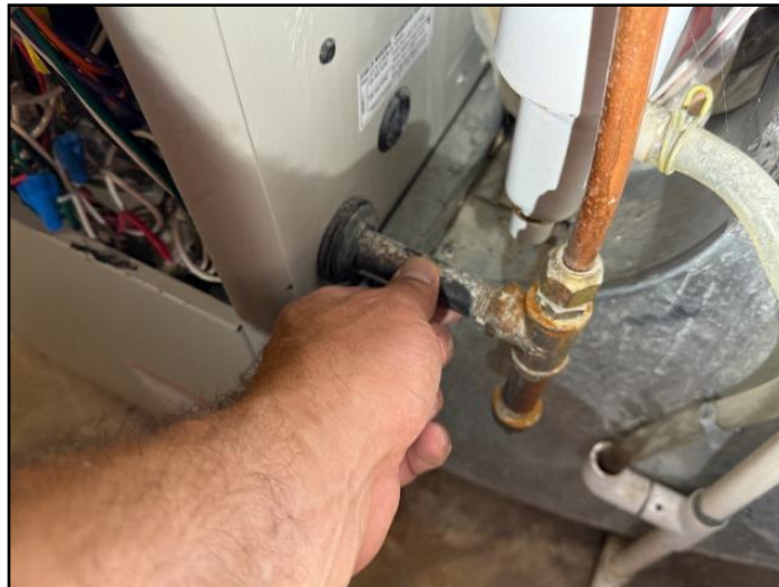
21. Inadequate support
