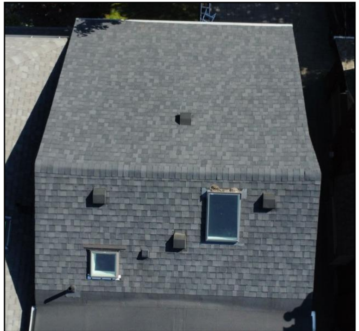
3. Asphalt shingles - at front home
