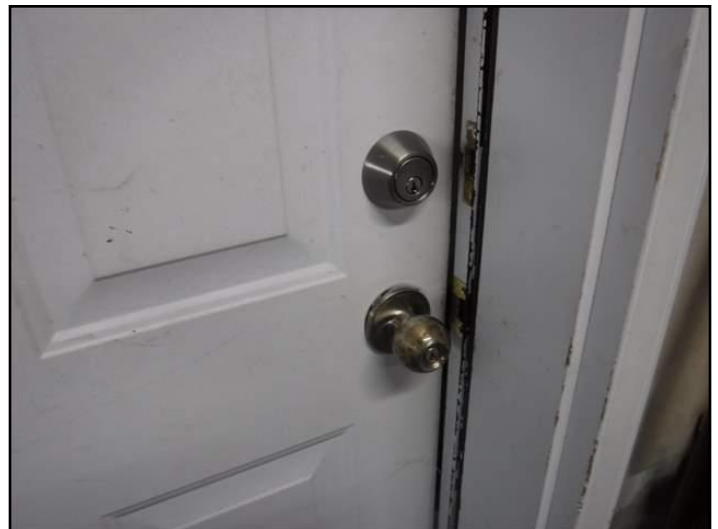
Does not fully latch
