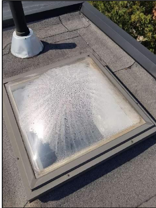
12. Lost seal on double glazing.
