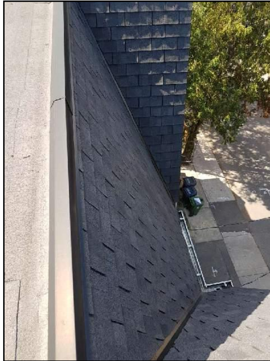
1. Asphalt shingles
