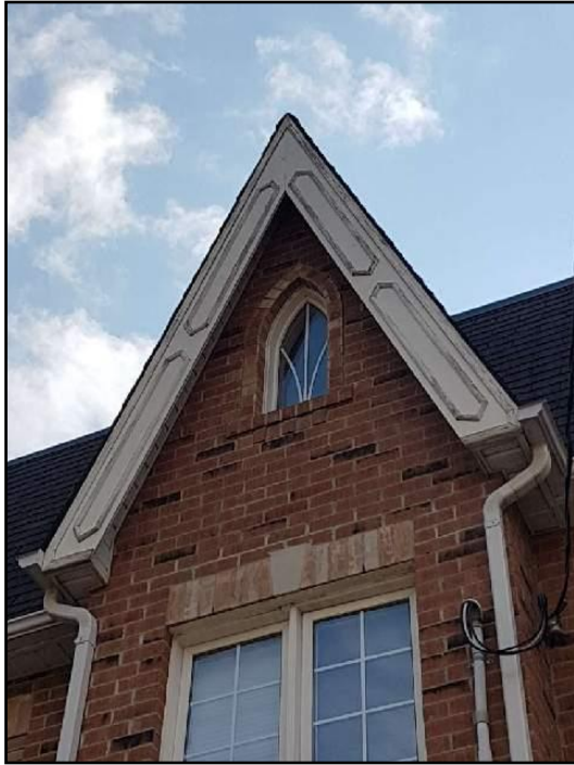
4. Paint - deteriorated / missing
