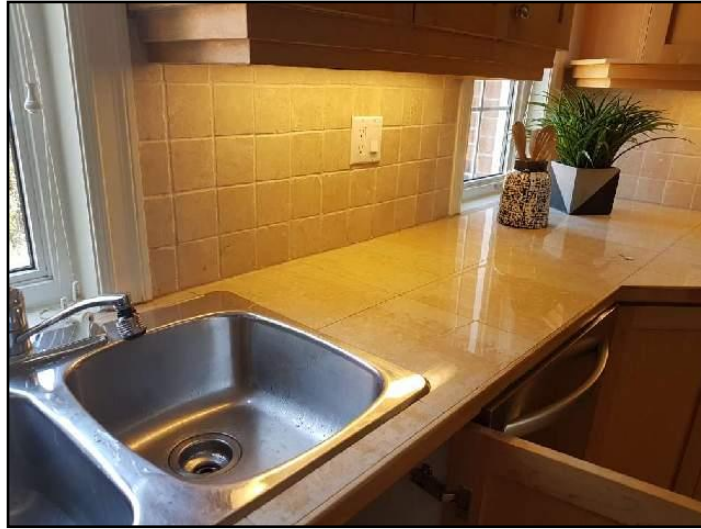
7. GFCI/GFI needed (Ground Fault Circuit...
