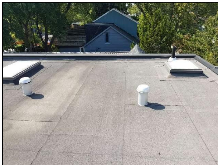
2. Modified bitumen membrane
