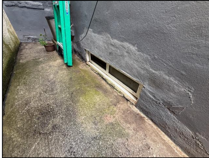
7. Sill - Near or at Grade Level
