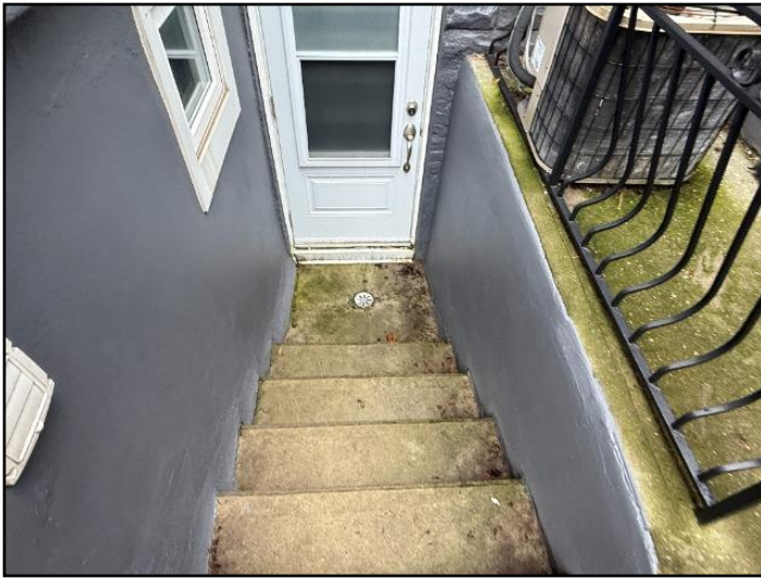
8. Missing handrail
