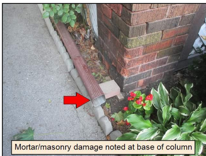
Discharge too close to Column / Post...
