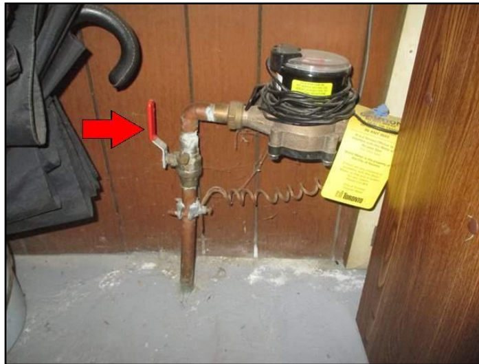
Main water shut-off valve
