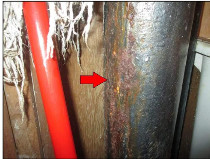
The cast iron waste piping is near the end...
