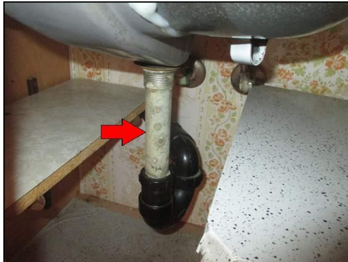
Tail piece corroded
