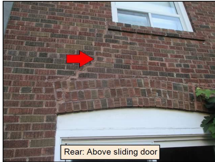
Example: Cracks/lateral movement
