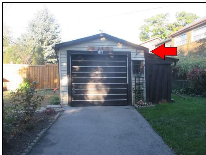
Structure out of plumb
