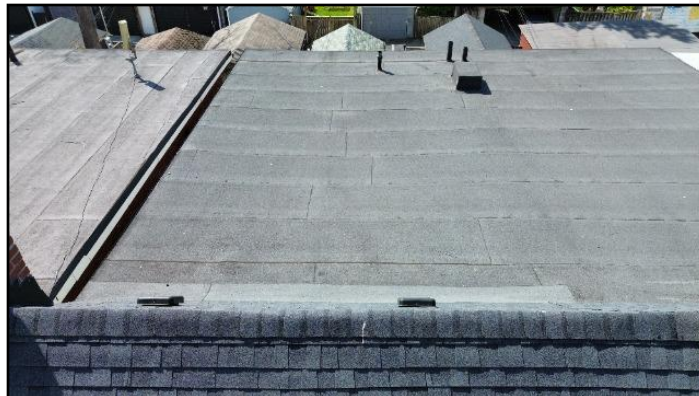
2. Modified bitumen membrane
