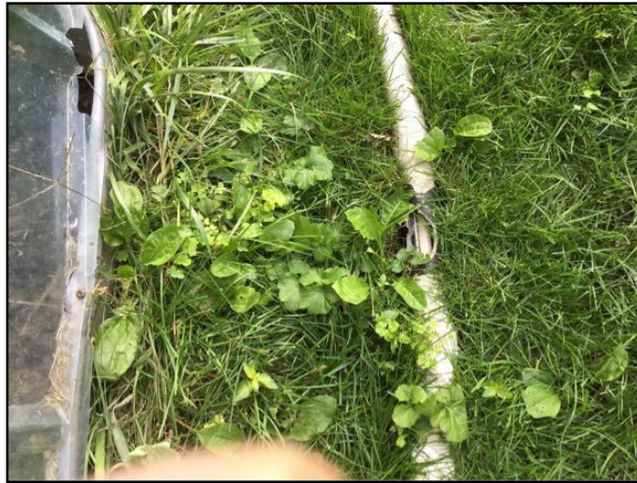
10. Damaged Conduct Implications Electric shock
