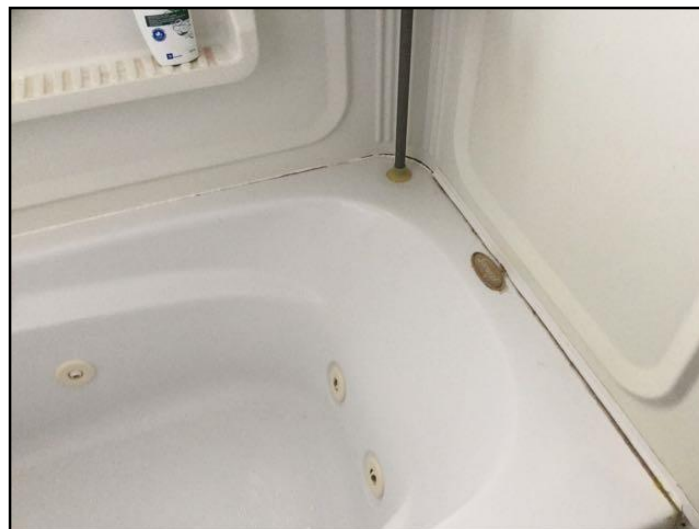
13. Caulking loose, missing or deteriorated
