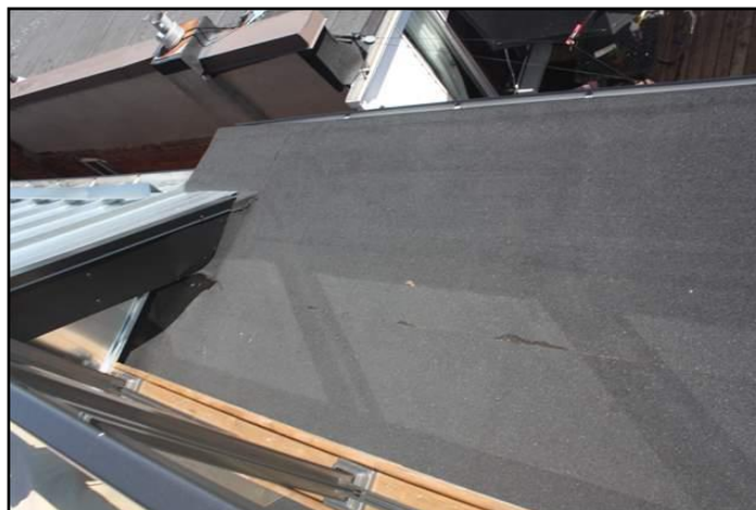
3. Modified bitumen membrane
