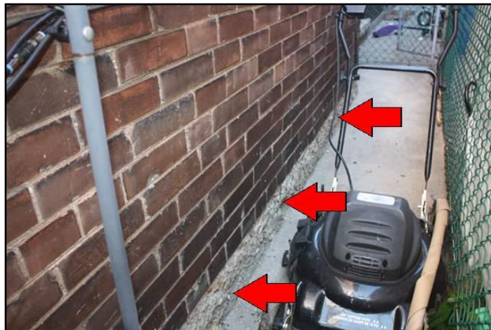
5. Parging damaged or missing
