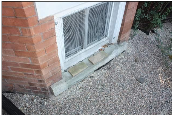
4. Sill deteriorated
