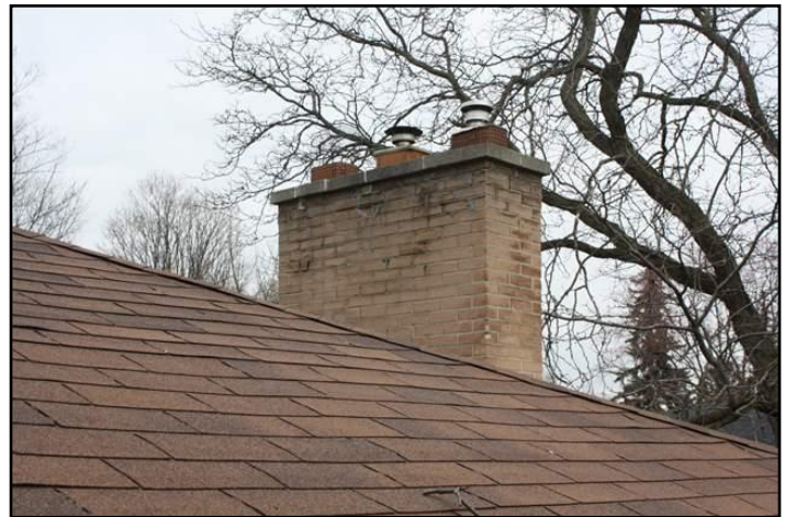
16. Loose, missing or deteriorated masonry
