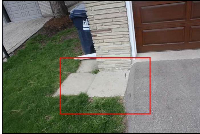
9. Improper slope or drainage
