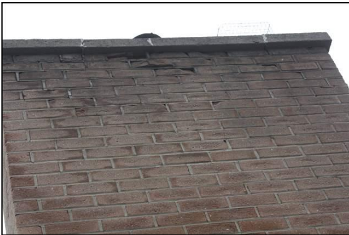
15. Loose, missing or deteriorated masonry
