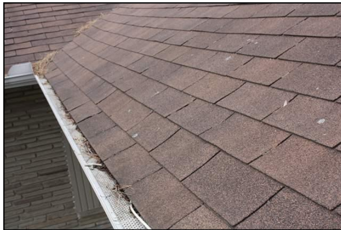
3. Asphalt shingles
