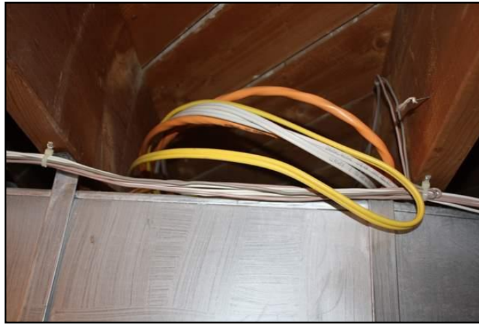
12. Too close to duct, pipe, vent or chimney
