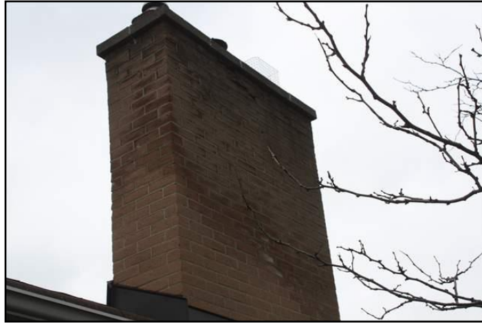
17. Loose, missing or deteriorated masonry
