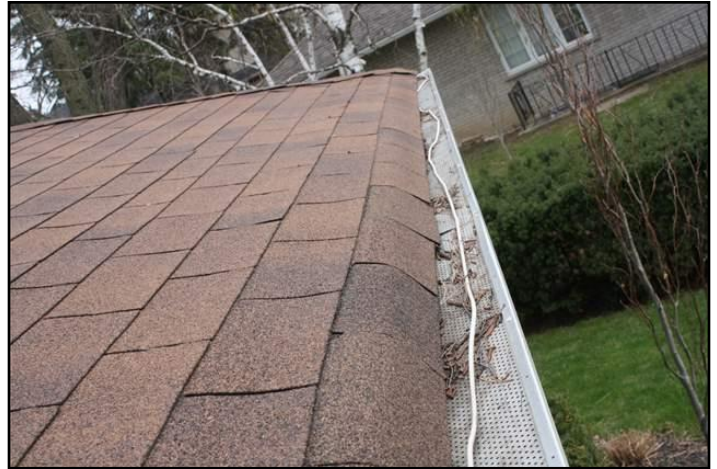
2. Asphalt shingles
