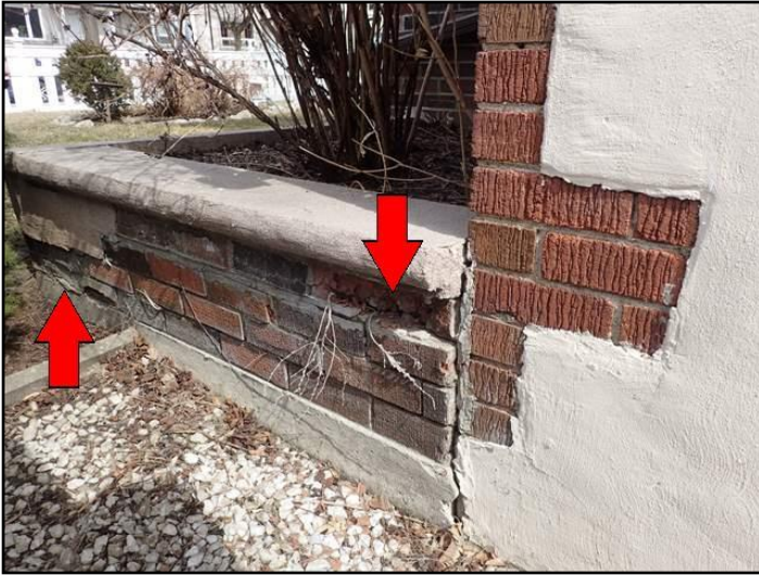
Masonry deterioration
