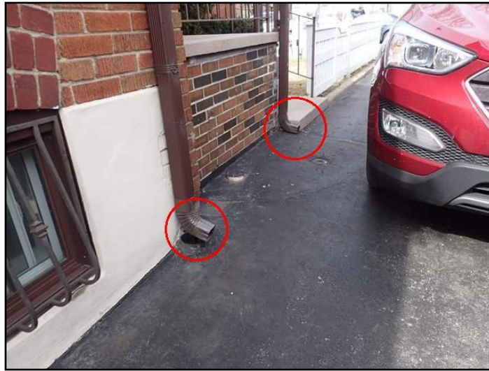
Less-than-ideal downspout location
