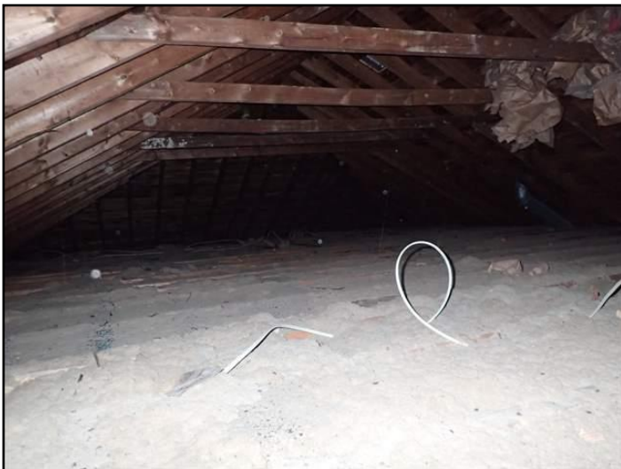
Insulation level less than current standards
