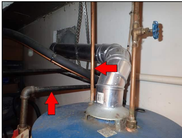
Bonding (for Gas Piping) - missing
