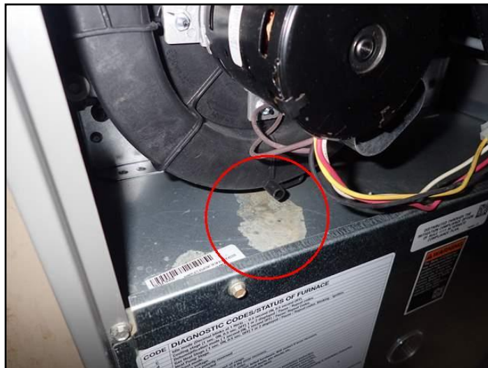
Water stains in cabinet (dry at inspection)
