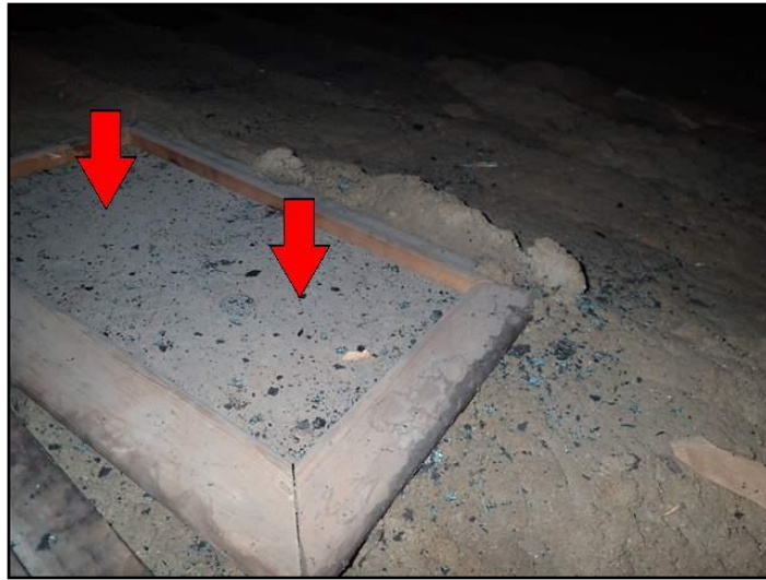
Attic access hatch not insulated
