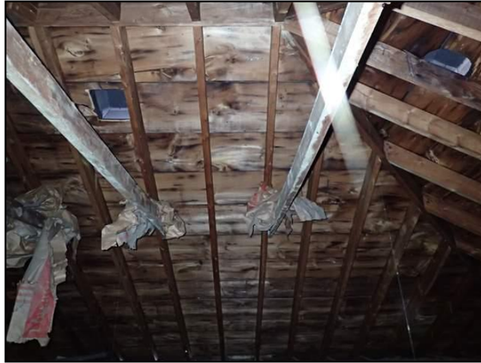
Roof sheathing is in good condition
