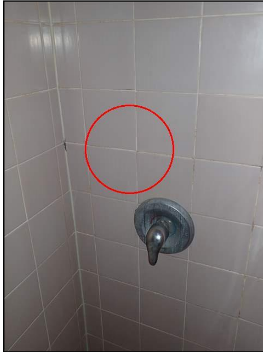
Loose, displaced tile in Basement shower
