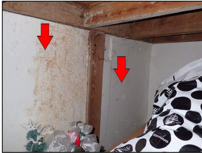
Exposed combustible insulation
