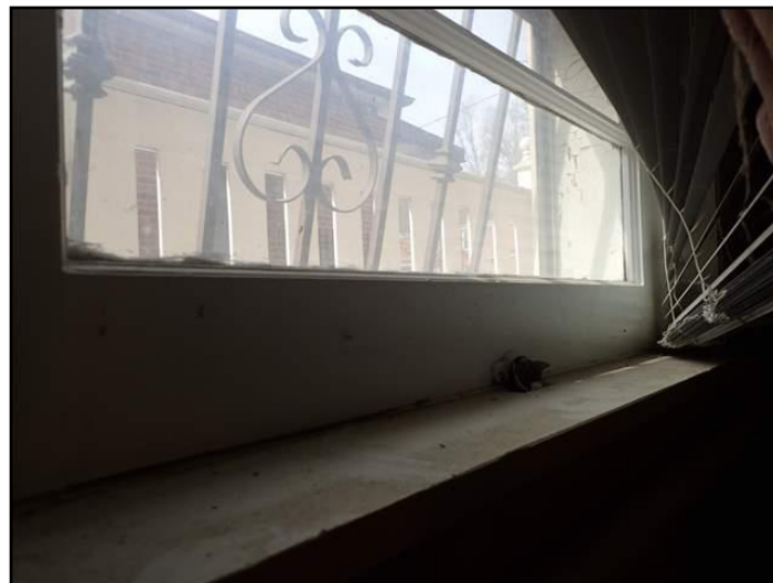
Window painted shut in Basement
