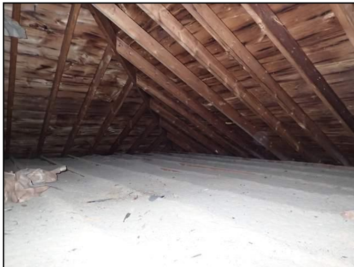
Insulation is evenly distributed
