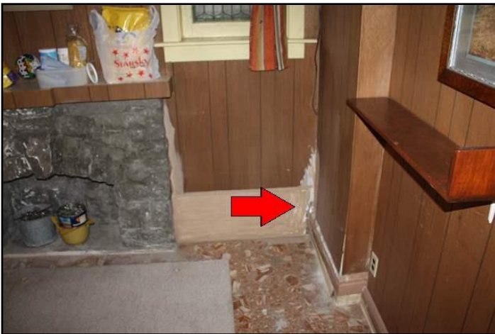
25. Dampness on floor or walls
