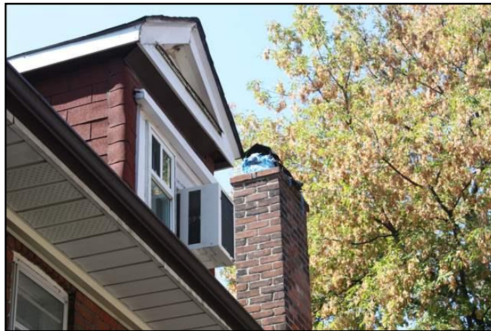
12. Loose, missing or deteriorated masonry
