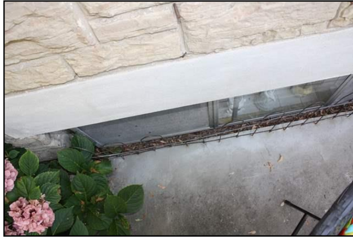
6. Sill - Near or at Grade Level
