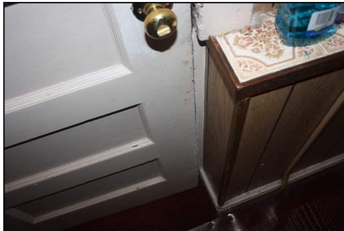
19. Loose or poor fit
