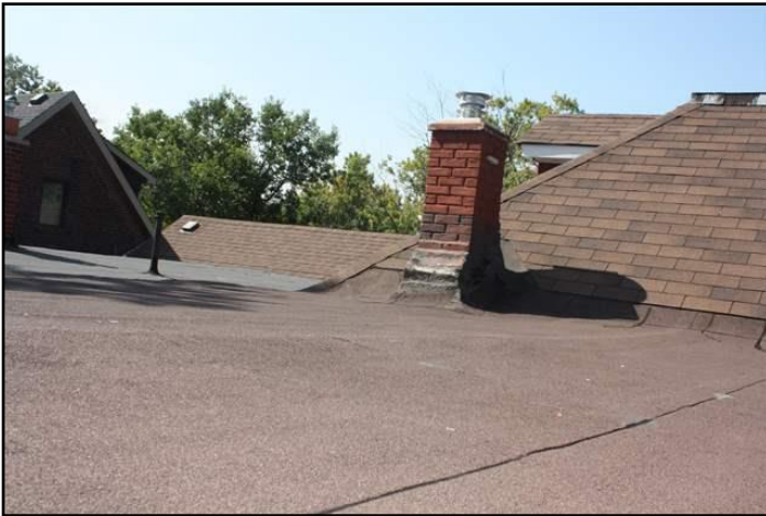
1. Modified bitumen membrane
