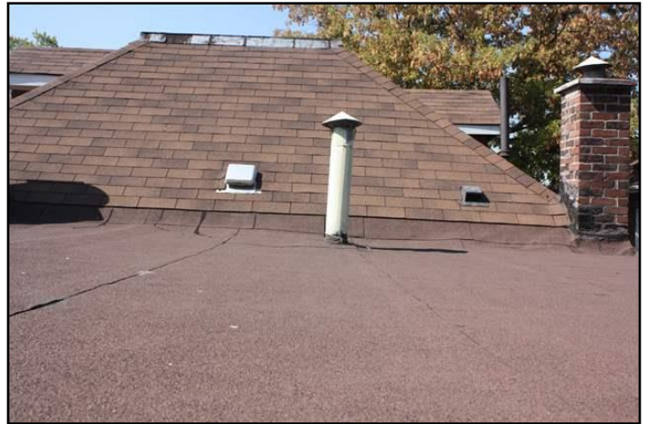
2. Modified bitumen membrane
