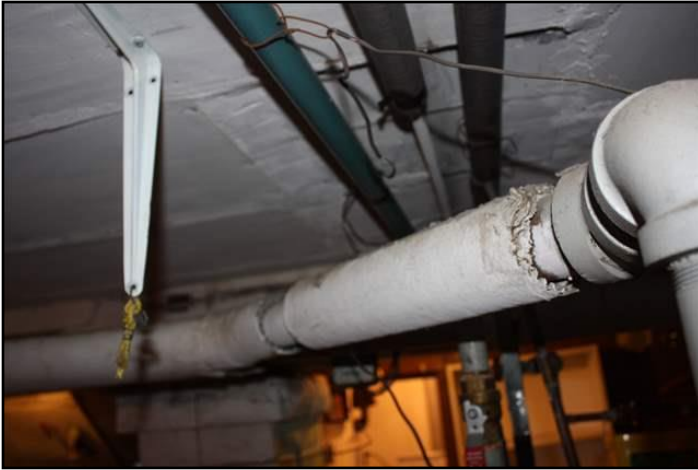
10. The insulation on the boiler or heating...
