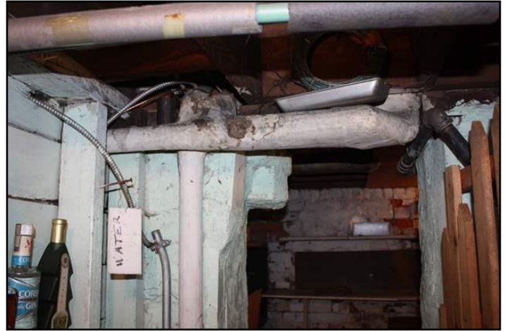
11. The insulation on the boiler or heating...
