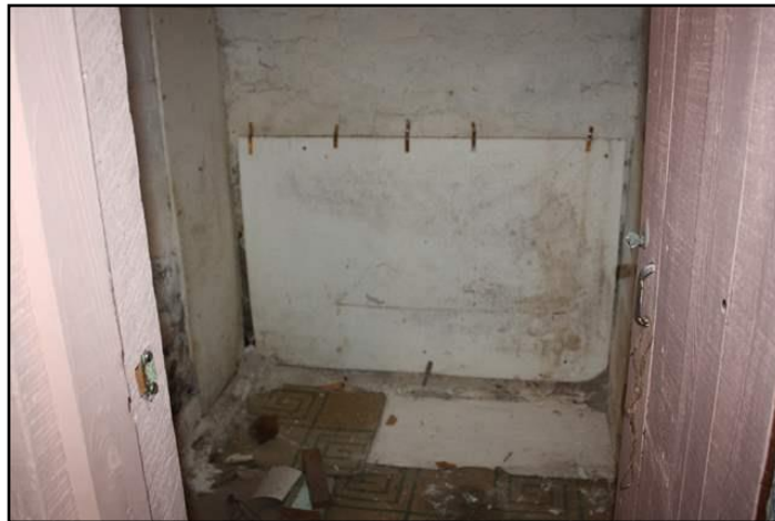
13. Exposed combustible insulation
