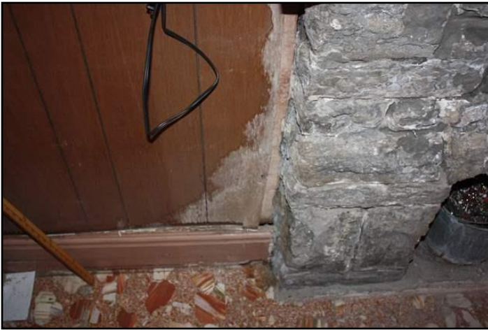
23. Dampness on floor or walls
