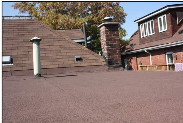
3. Modified bitumen membrane
