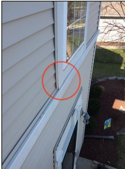
11. Caulking missing or ineffective
