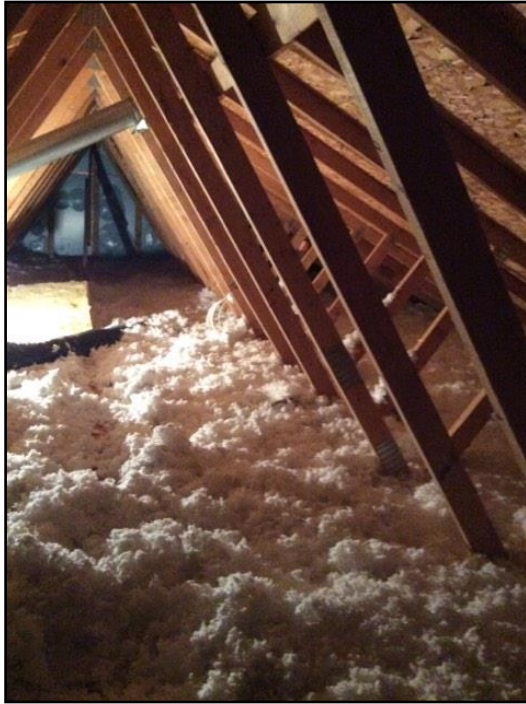
19. Rafters/roof joists
