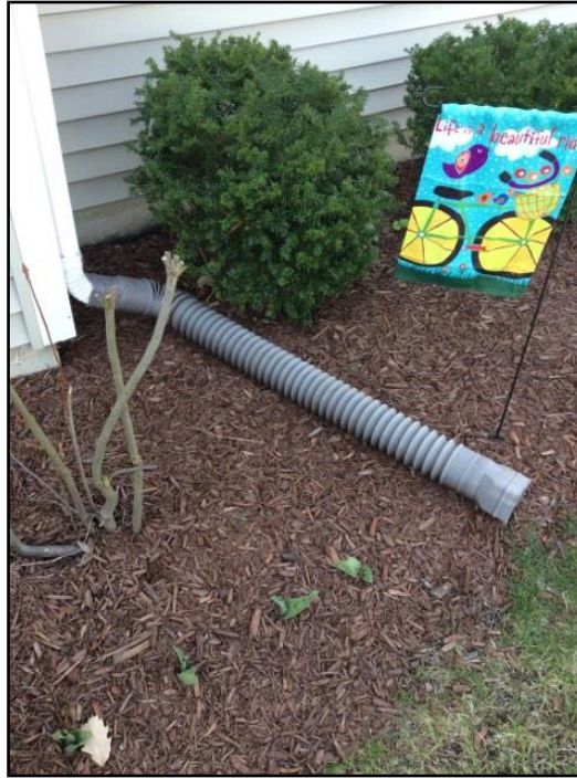
9. Should discharge 6 feet from building
