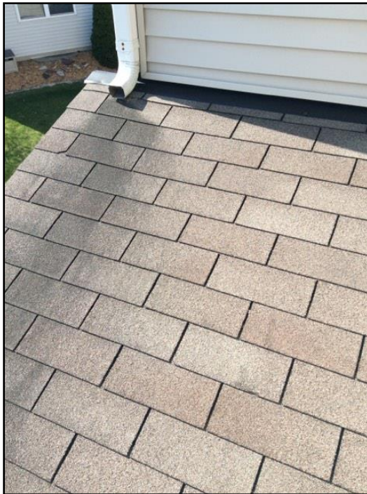
7. Downspouts discharging onto roofs
