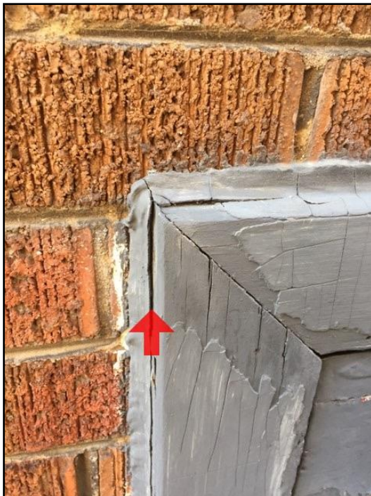
Caulking missing or deteriorated
