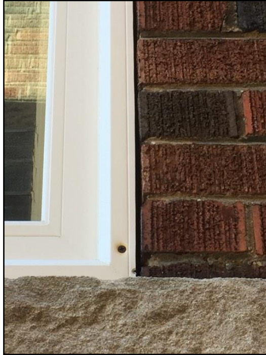
Caulking missing, loose or deteriorated
