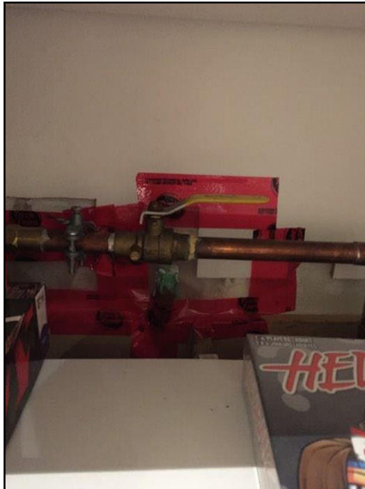
Water shut-off valve
