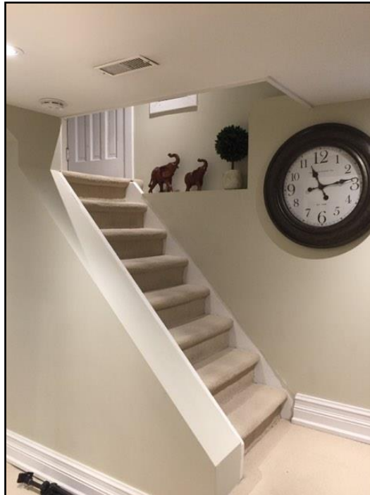
Missing guardrail
