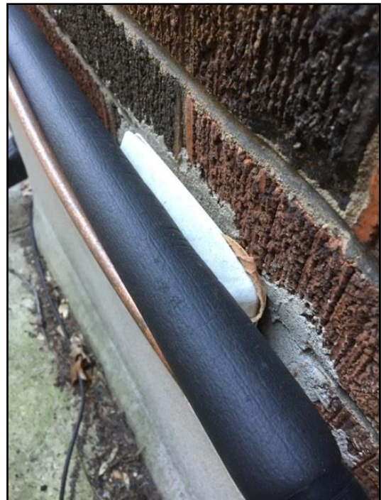
Caulking missing or deteriorated
