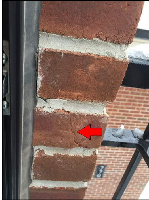
Minor Brick Damage
