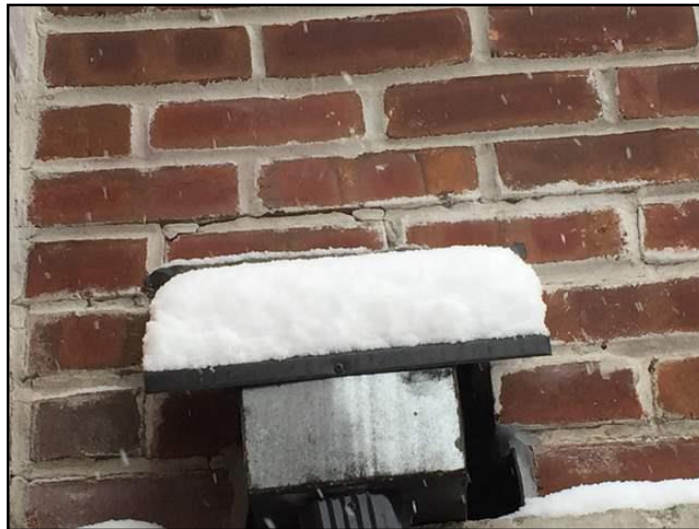
Example of minor cracks
