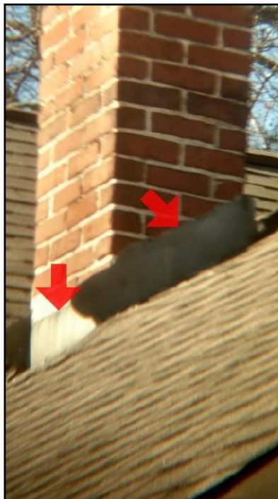
3. Not let into mortar joints
