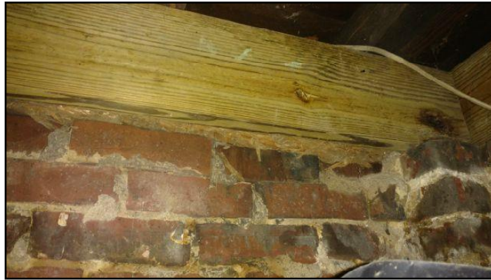
28. Rot or insect damage
