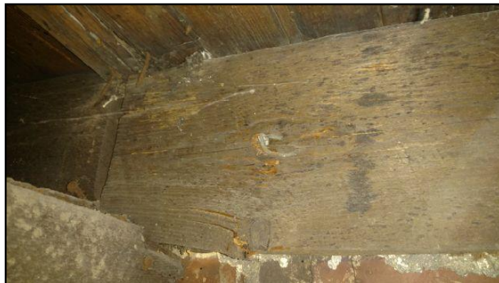
30. Rot, insect or fire damage
