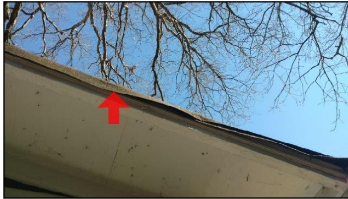
1. Overhangs too big or small Asphalt roofing...
