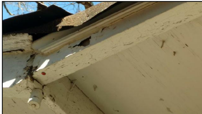
5. Water Damaged
