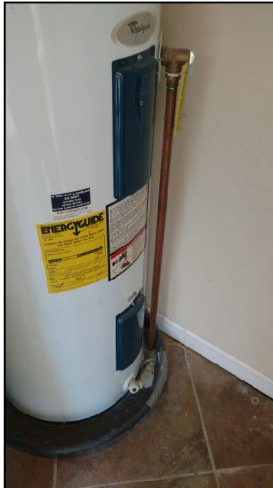
51. TPR Drainline draining in to pan instead of...
