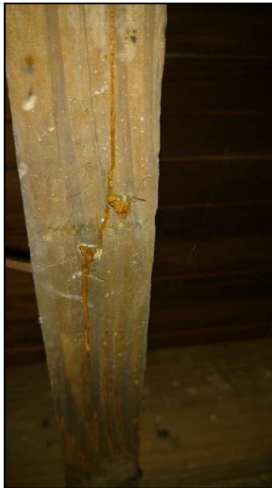
39. Rot, insect or fire damage
