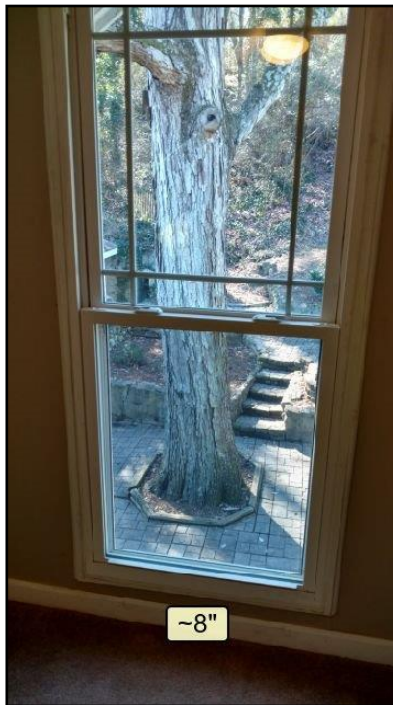
59. Safety glass not installed
