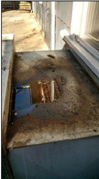
48. Cowling is sagging and retaining water and...
