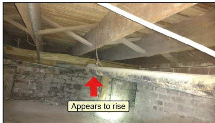
52. Fall on drain line is not sufficient
