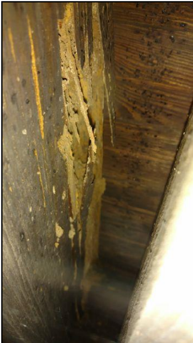
31. Rot, insect or fire damage
