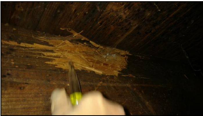
37. Rot, insect or fire damage
