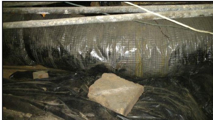
47. Ductwork is laying on the ground. This will...
