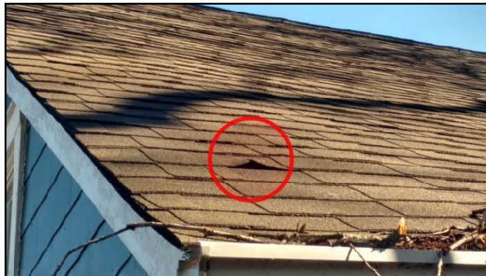
2. Raised fasteners under roofing - When you...
