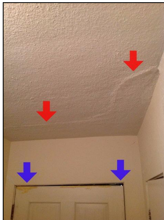
55. Crack and door reveal
