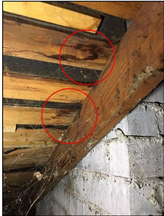
43. Evidence of past leakage under chimney
