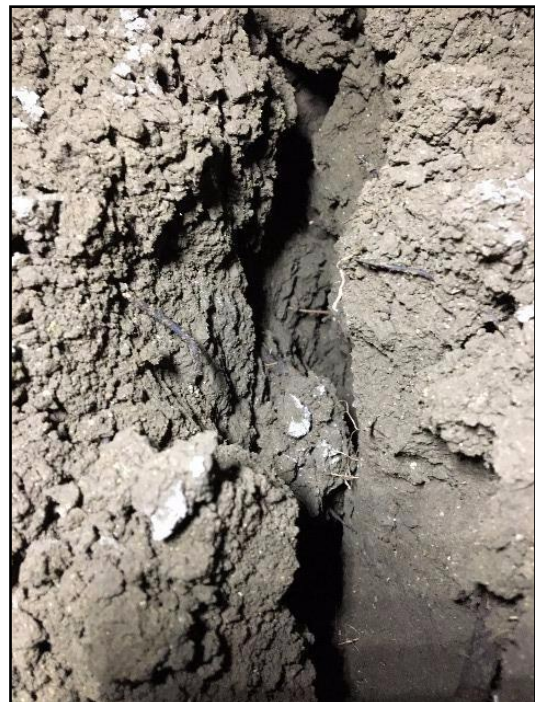
58. Expansive Soil - large crack found under home
