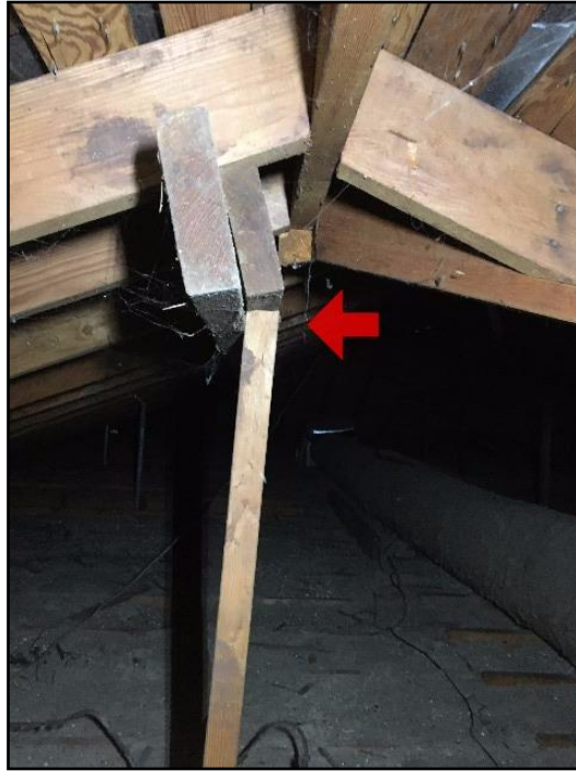
74. Poor connections
