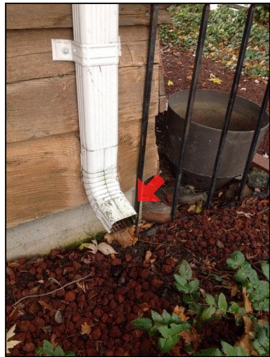
8. Downspouts end too close to building
