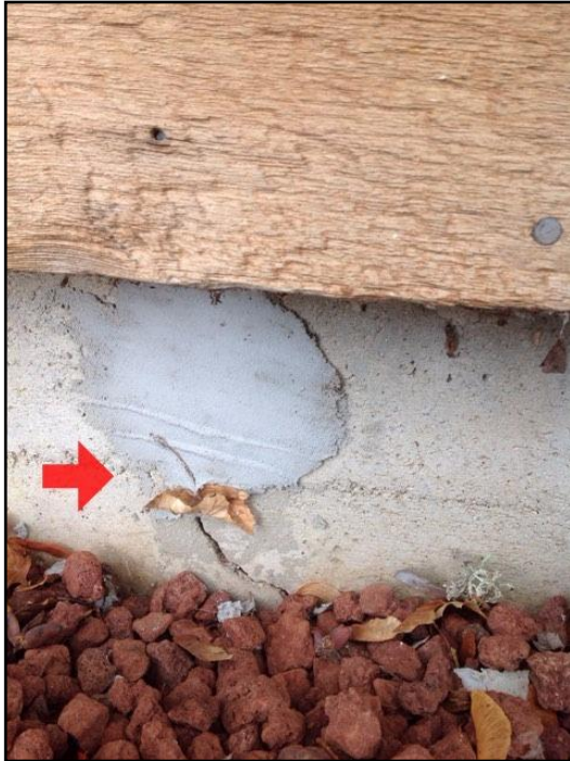
20. Typical minor cracks
