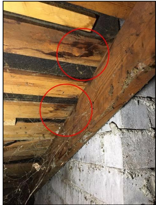
5. Evidence of past leakage under chimney
