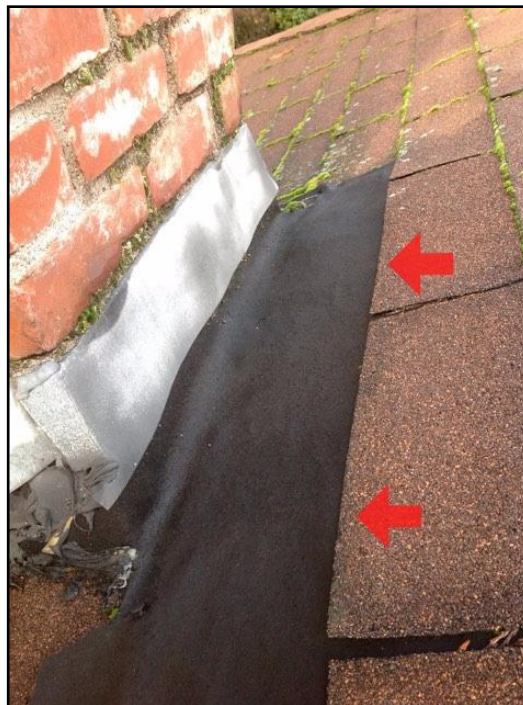
41. Missing top, bottom, side flashings
