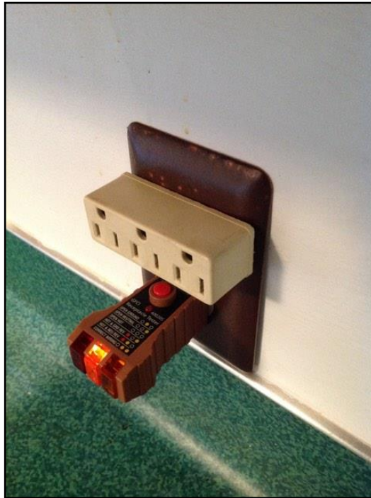
82. No GFCI Outlet in Kitchen
