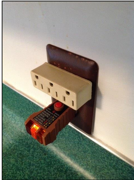
27. No GFCI Outlet in Kitchen
