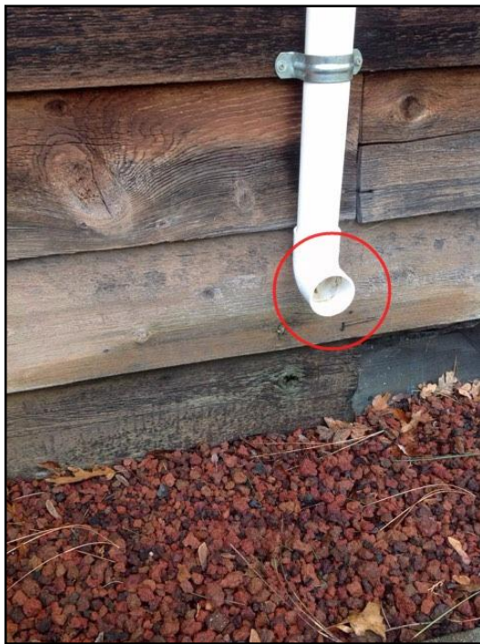
7. Downspouts end too close to building
