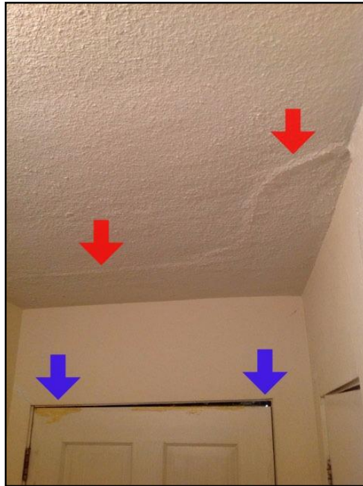
12. Crack and door reveal
