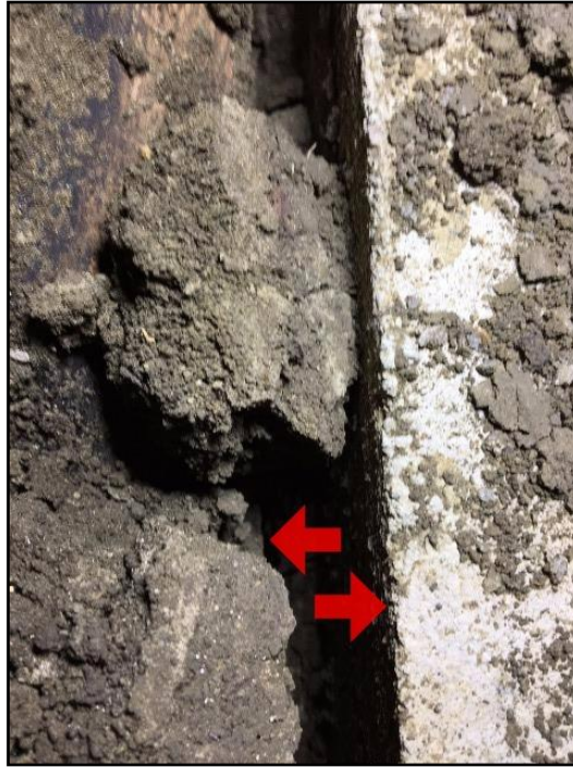
59. Evidence of movement - gap
