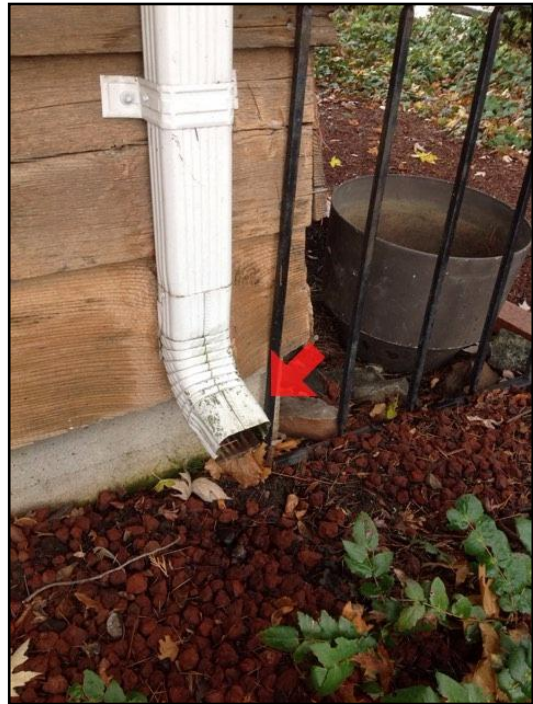
49. Downspouts end too close to building
