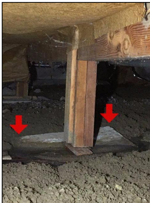
64. Footing movement and standing water
