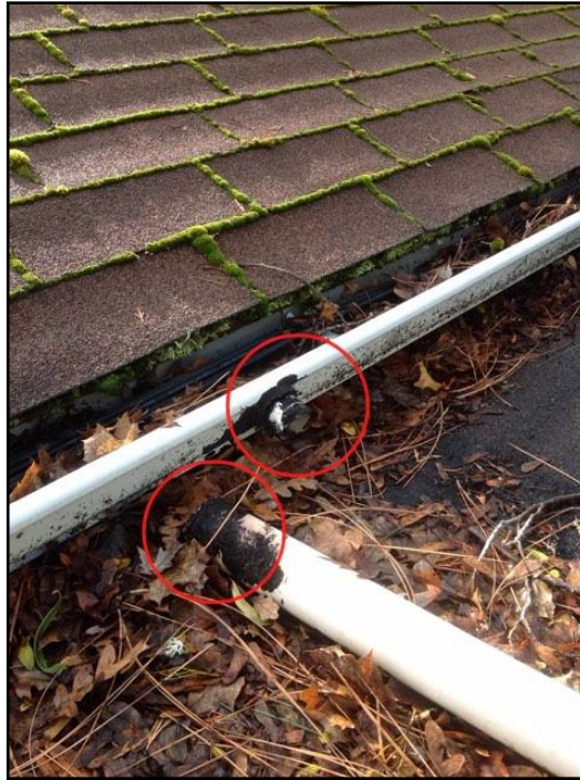
47. Discharging onto roof
