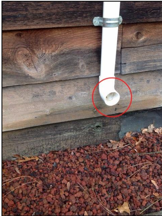
48. Downspouts end too close to building
