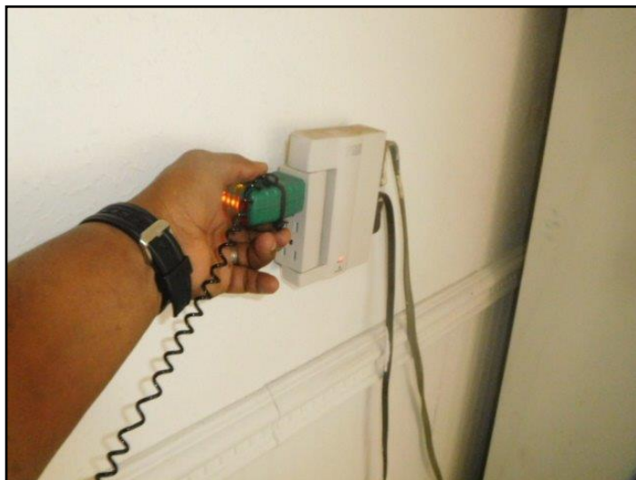
74. GFCI/GFI needed (Garage)
