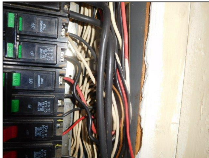
64. Box not bonded to ground
