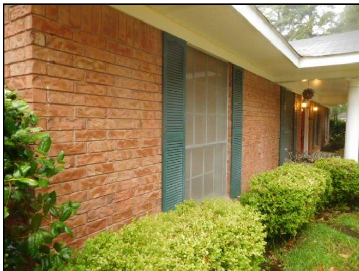
55. Wood frame / Brick veneer
