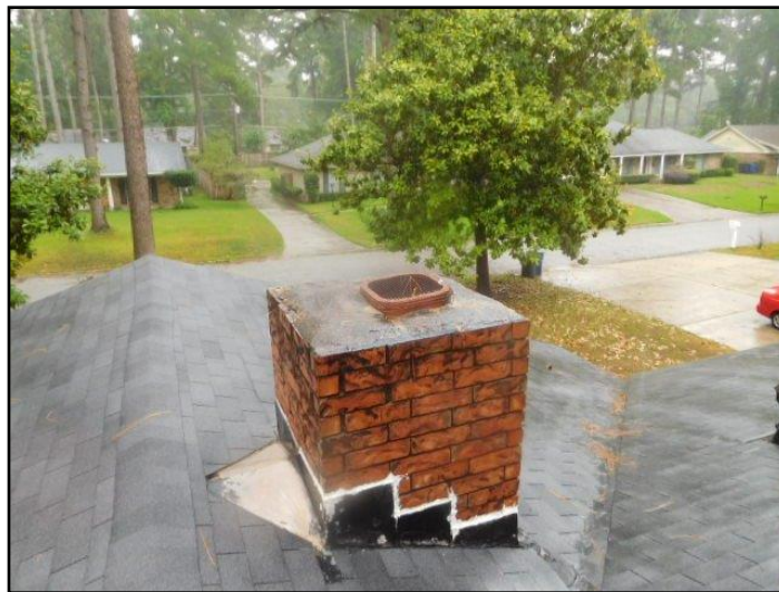
85. Missing chimney cap
