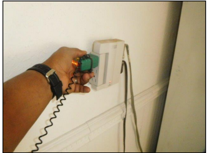
19. GFCI/GFI needed (Garage)
