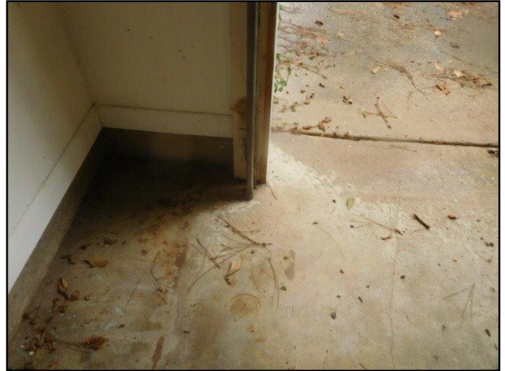
7. Missing auto reverse sensors
