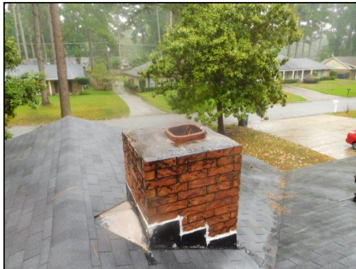
24. Missing chimney cap
