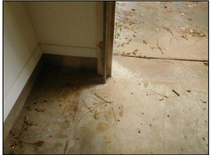
52. Missing auto reverse sensors
