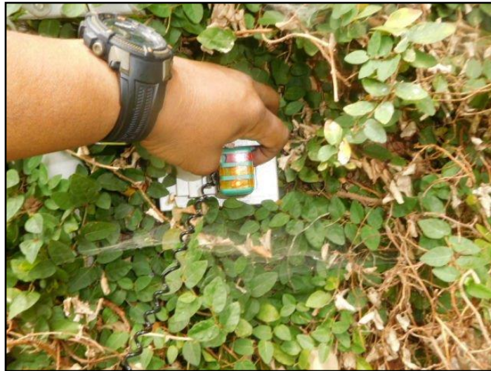
77. GFCI/GFI needed (Exterior)
