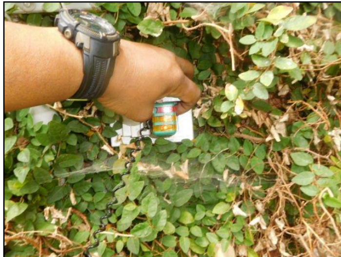
22. GFCI/GFI needed (Exterior)
