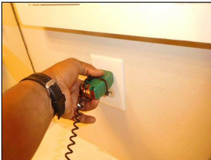
73. GFCI/GFI needed (Master Bath)
