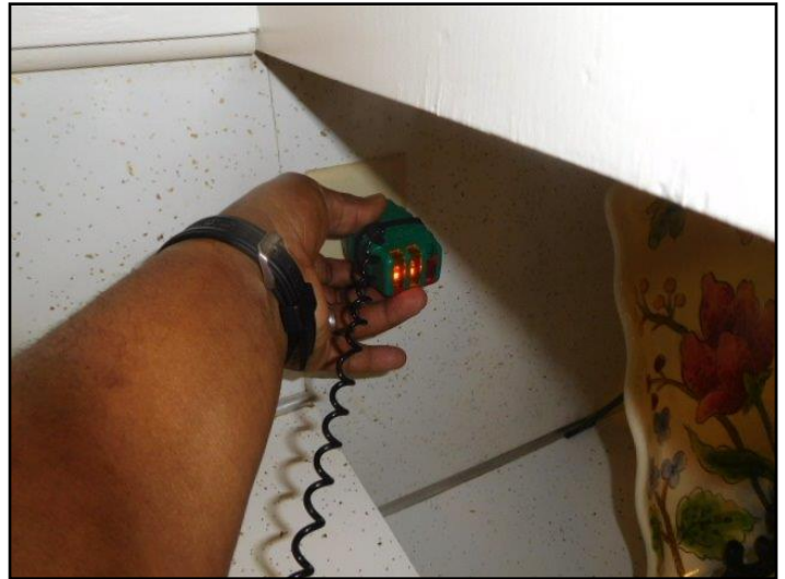
76. GFCI/GFI needed (Kitchen)ircuit...
