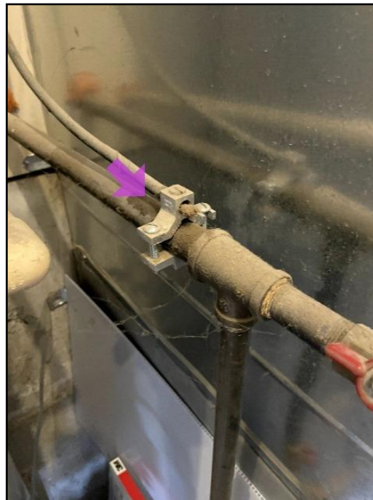
21. Gas bonding location
