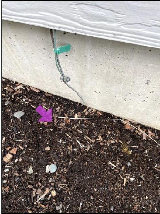
19. Copper - water pipe and ground rod
