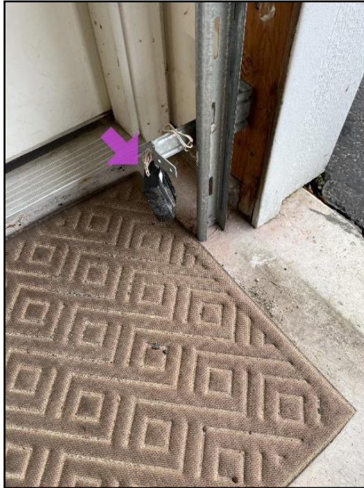
7. Sensors damaged
