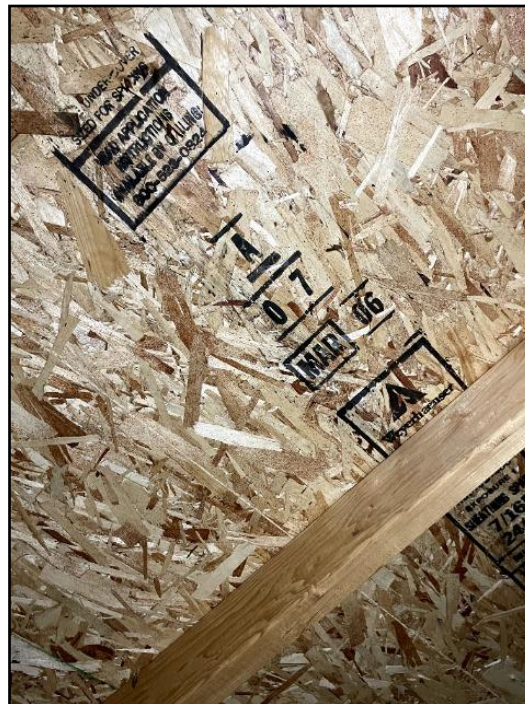
16. Oriented Strand Board (OSB) sheathing
