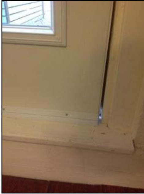
43. Weatherstripping missing or ineffective
