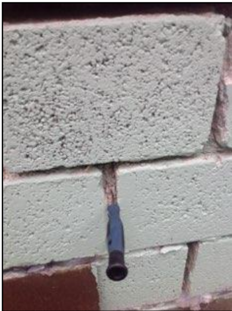
35. Loose, missing or deteriorated masonry
