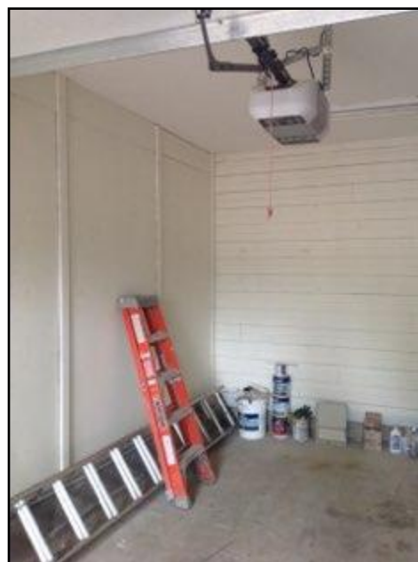
52. Fire separation between garage and living...
