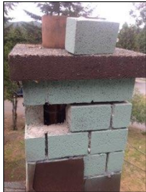
36. Loose, missing or deteriorated masonry
