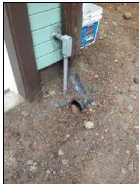
10. Downspouts end too close to building
