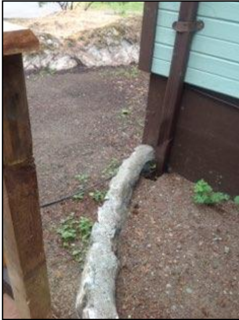
23. Missing extend rail
