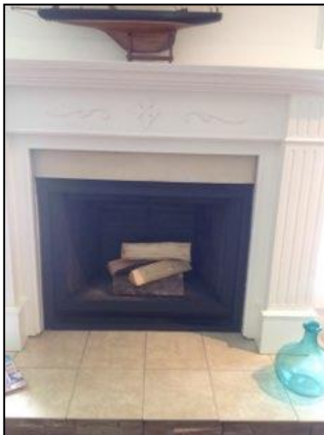
34. Inadequate clearance from combustibles
