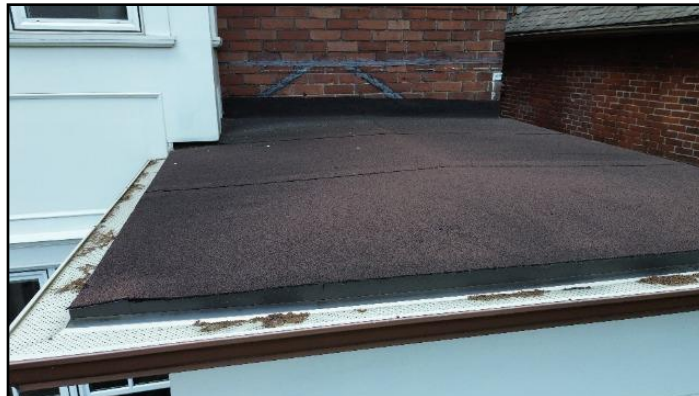
2. Modified bitumen membrane
