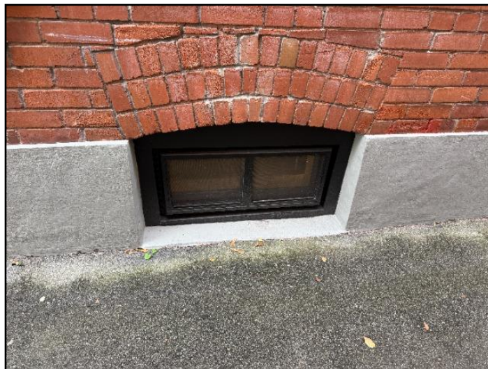
6. Sill - Near or at Grade Level
