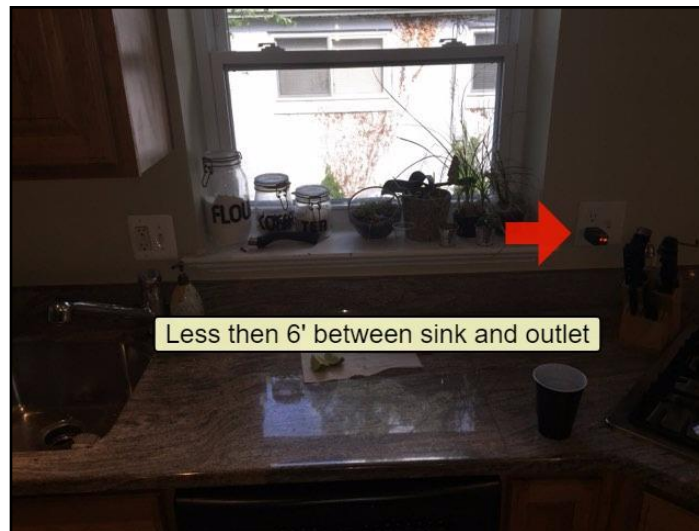
No GFCI/GFI (Ground Fault Circuit...
