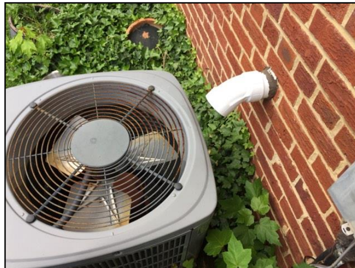
Poor vent location, arrangement
