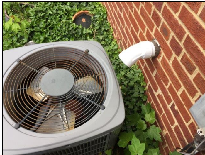
Poor vent location, arrangement
