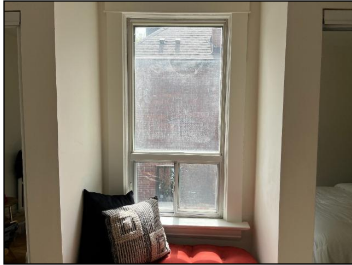
33. Lost seal on double or triple glazing
