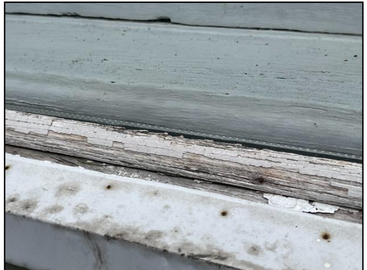
11. Paint and Caulking - deteriorated / missing
