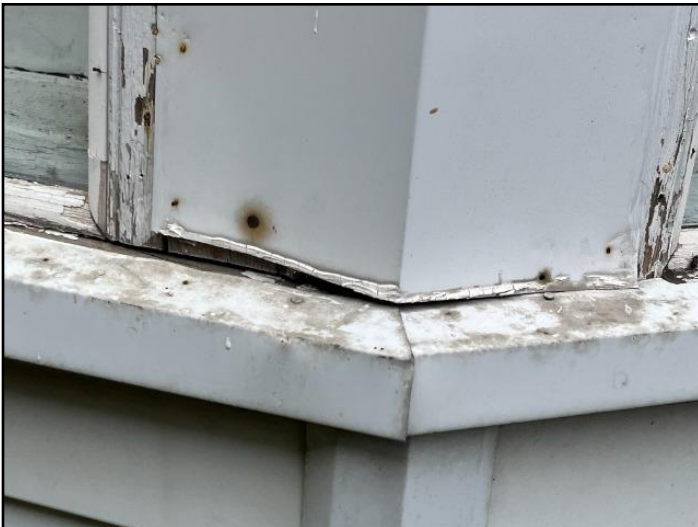
10. Paint and Caulking - deteriorated / missing
