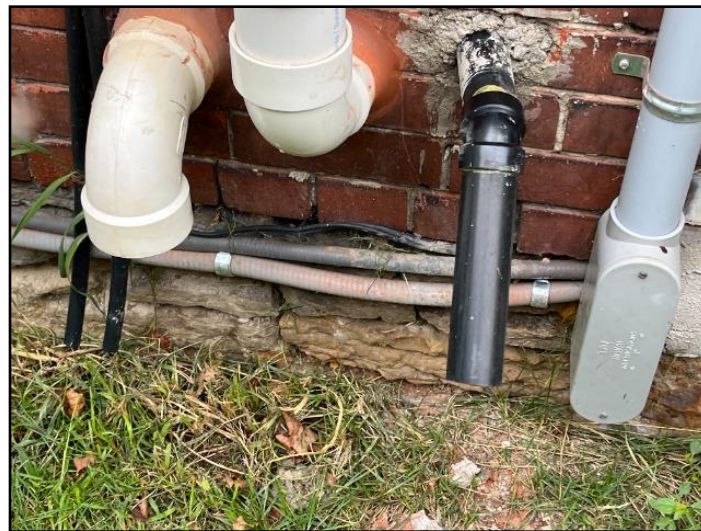
30. Discharges less than 6 feet from home
