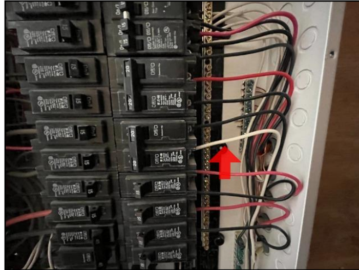
26. White wires connected to breakers not...
