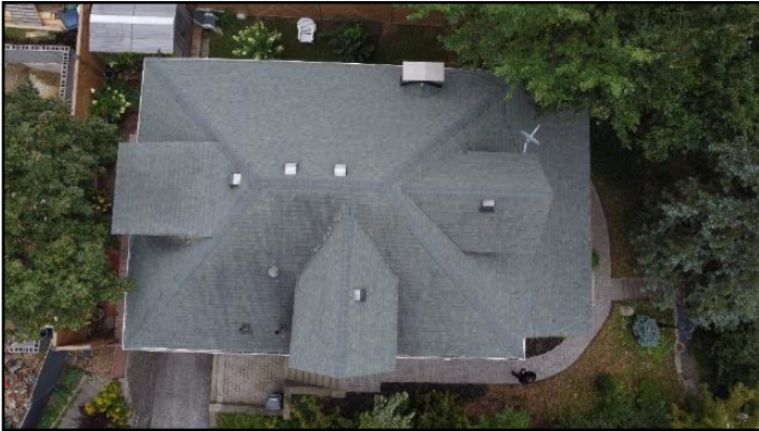
1. Asphalt shingles
