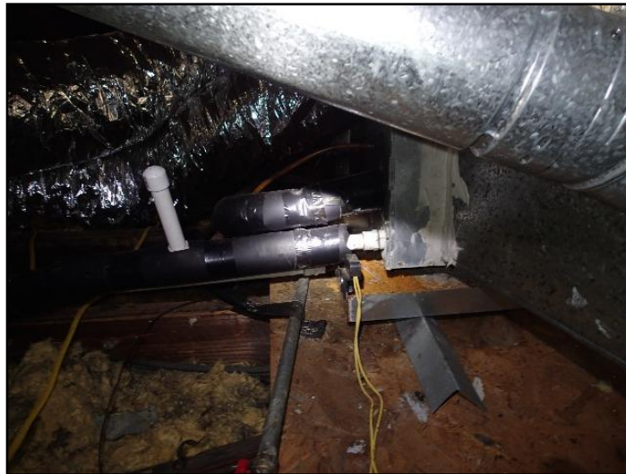
59. Float switch in pan.
