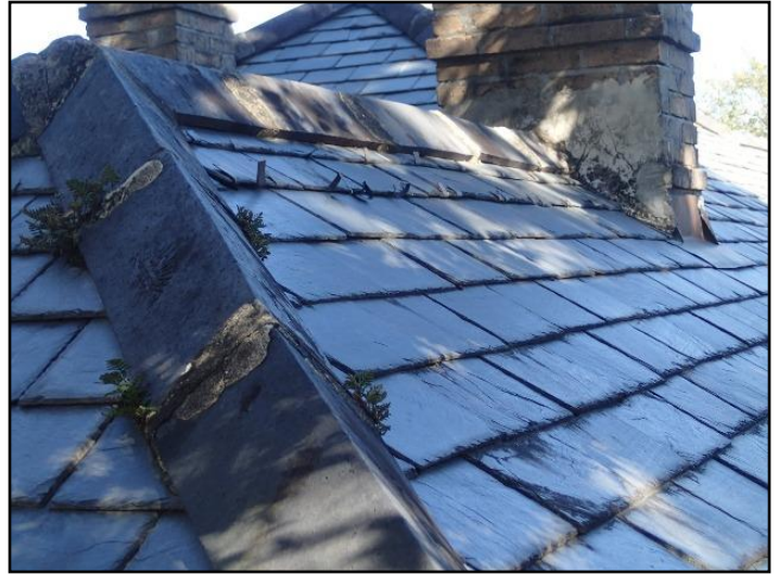
5. Prior repairs and moss/plant growth
