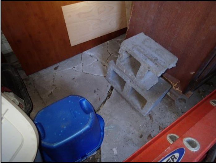
16. Broken concrete/Raised floor
