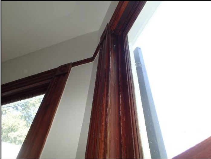
89. Broken / Missing sash cord/spring
