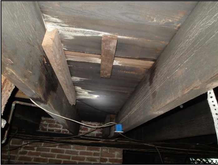
41. Prior repair from below
