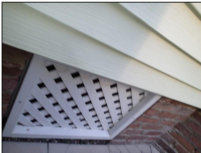
68. Lattice or barrier preventing access.
