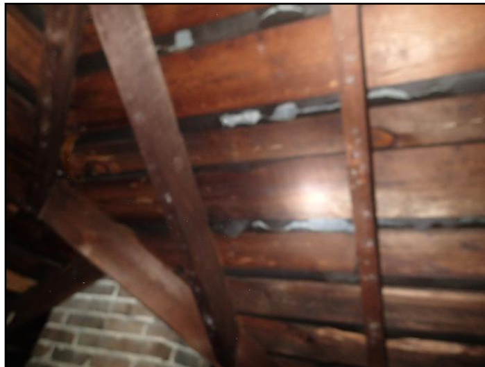
10. Torn / missing underlayment
