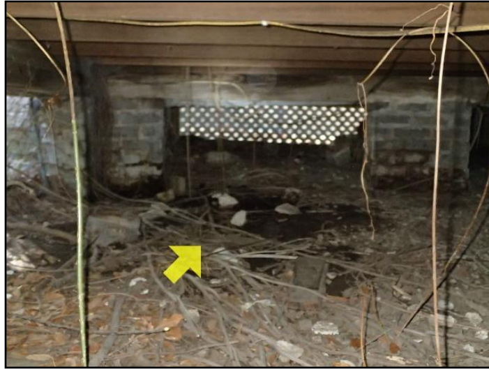
34. Improper slope or drainage
