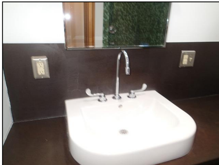
49. GFCI outlet on same circuit downstream of...
