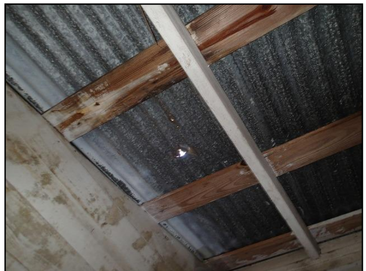
15. Hole in roof
