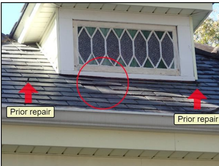
2. The slate roof appeared mostly functional a...
