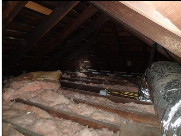
66. Glass fiber - Batts
