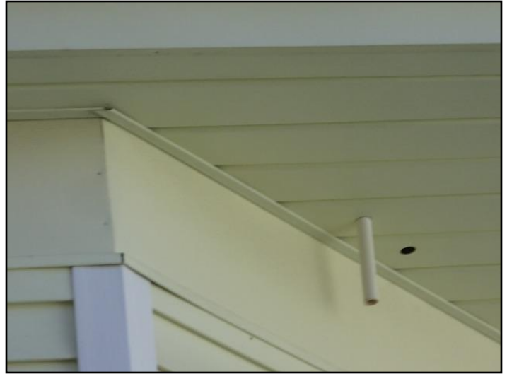
27. Opening in soffit
