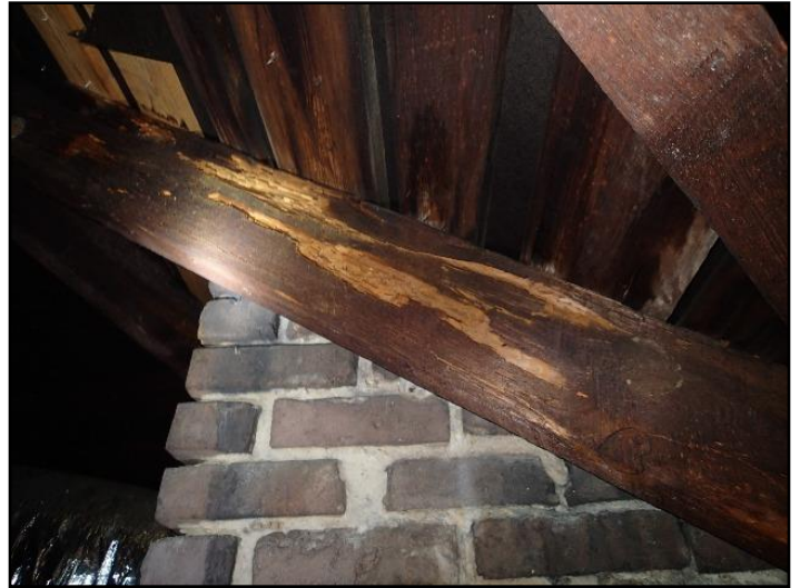
38. Damaged rafter
