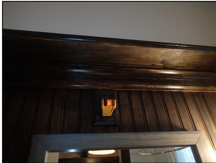
48. Ungrounded GFCI outlet
