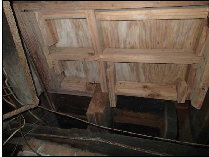
54. Floor furnace supported from below.
