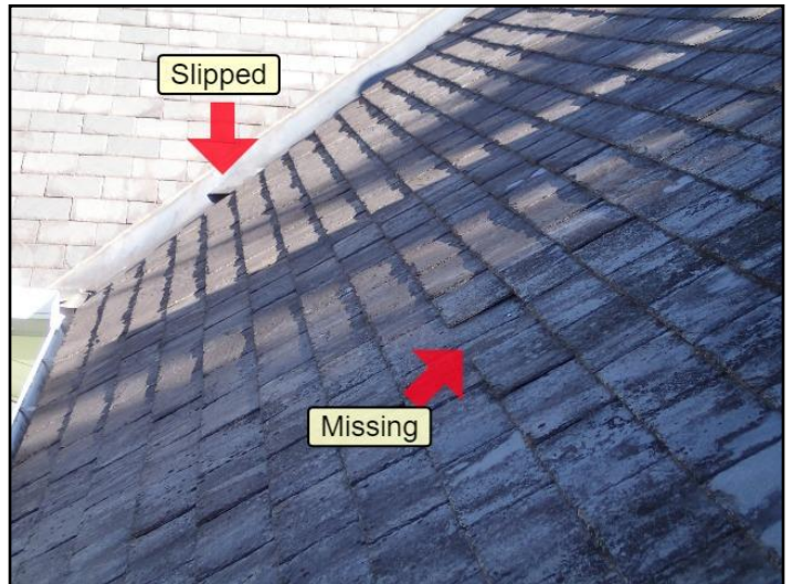
7. Missing tile & slipped tile
