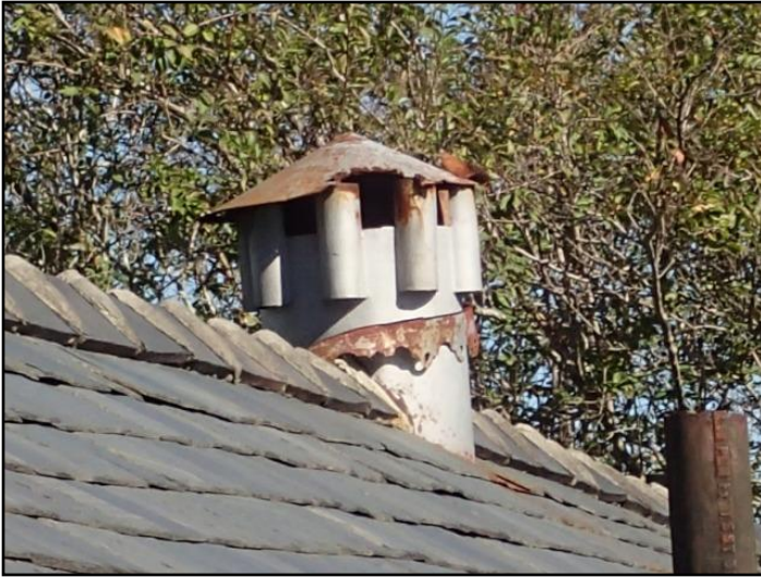
4. Rusted roof vent
