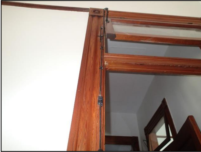
93. Missing latching hardware
