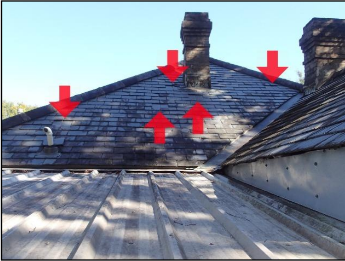
8. Slipped/missing tile
