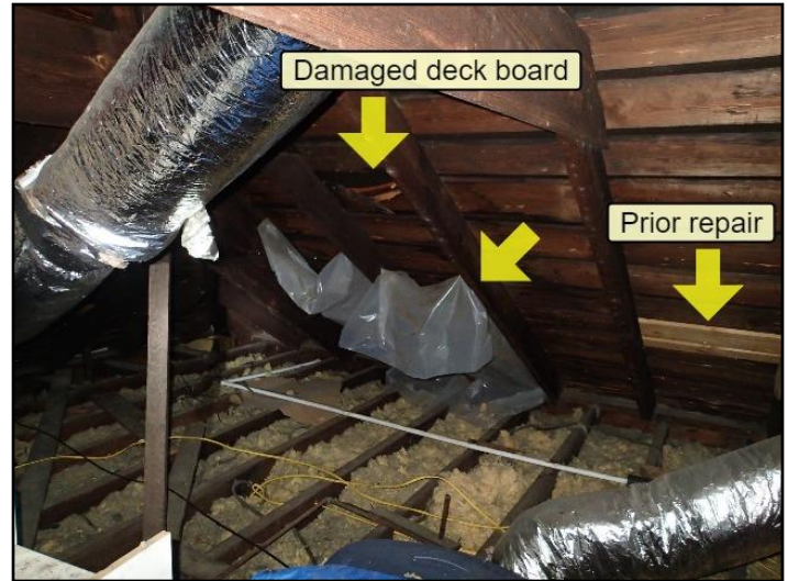
9. Plastic secured to rafters
