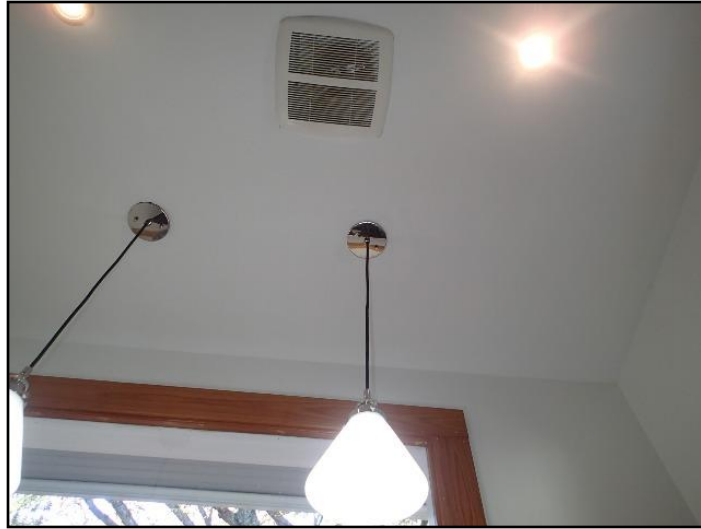
62. Missing AC register
