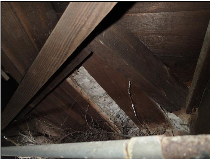
39. Damaged subfloor under fireplace
