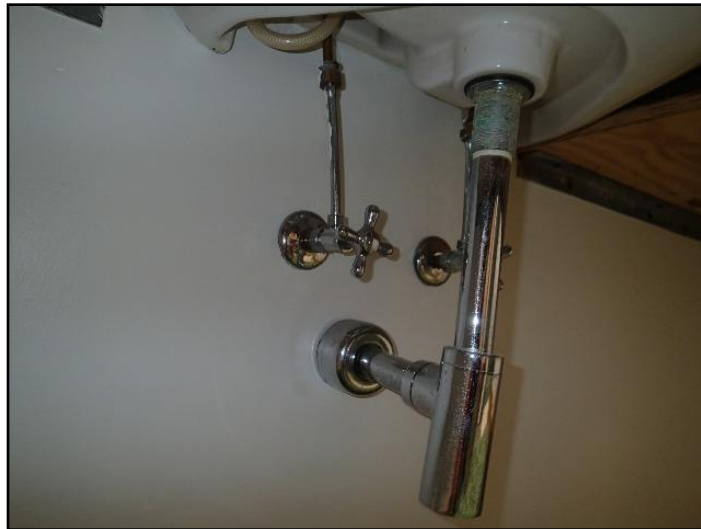
80. Bottle trap. Primary bathroom
