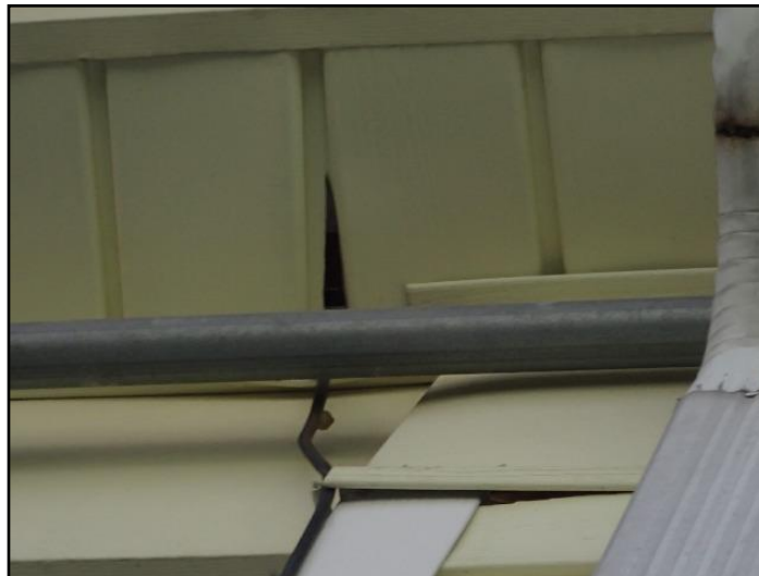
28. Opening in soffit
