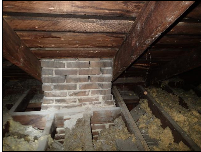
56. Missing or deteriorated masonry
