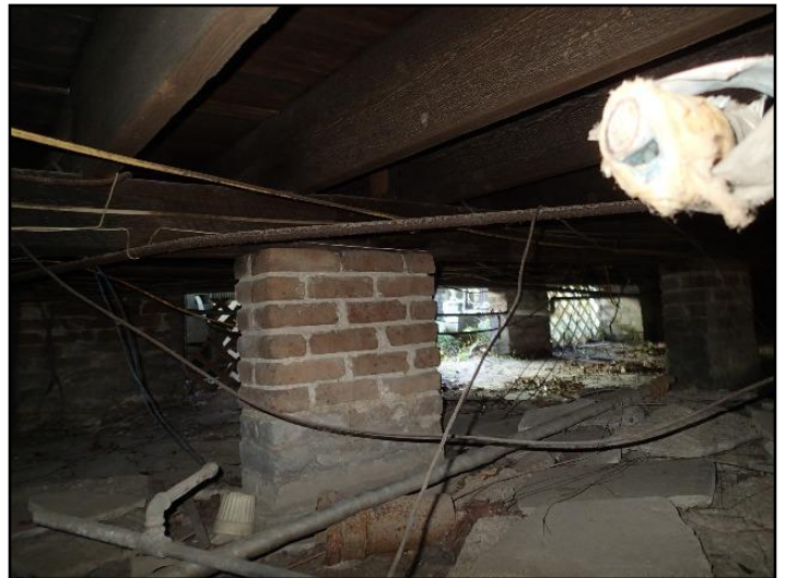
40. Missing mortar on piers.
