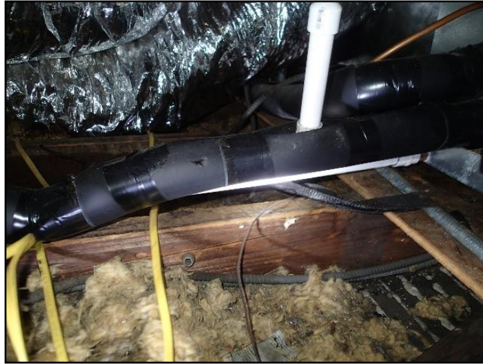
60. The condensate drain line has no float switch
