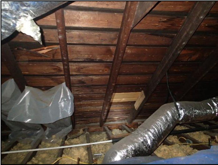
37. Prior repair to roof decking
