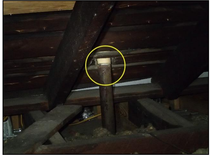
82. Not connected in attic
