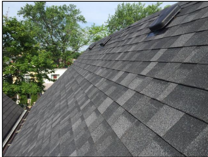
Asphalt shingles
