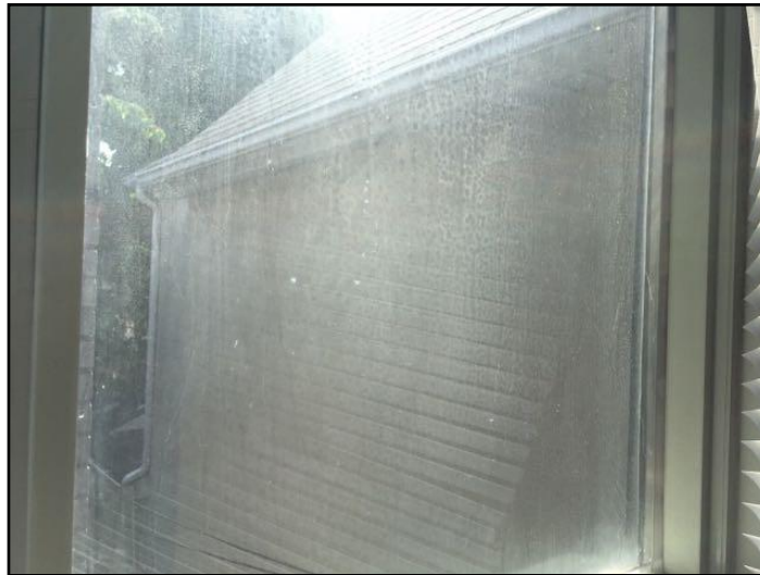
Lost seal on double or triple glazing
