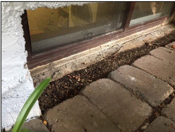
Window close to grade in well. Increase...
