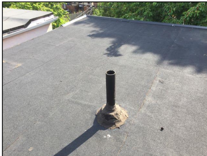
Modified bitumen membrane
