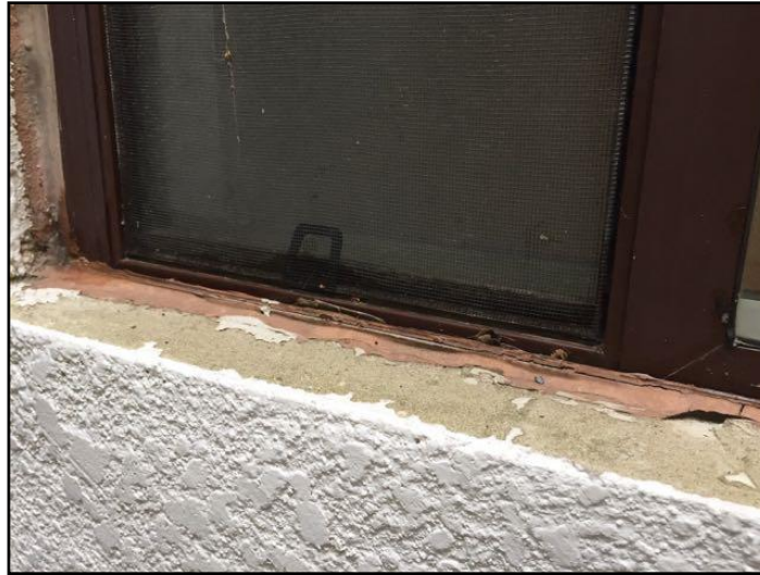
Caulking deteriorated
