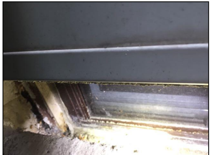
Window close to grade in well
