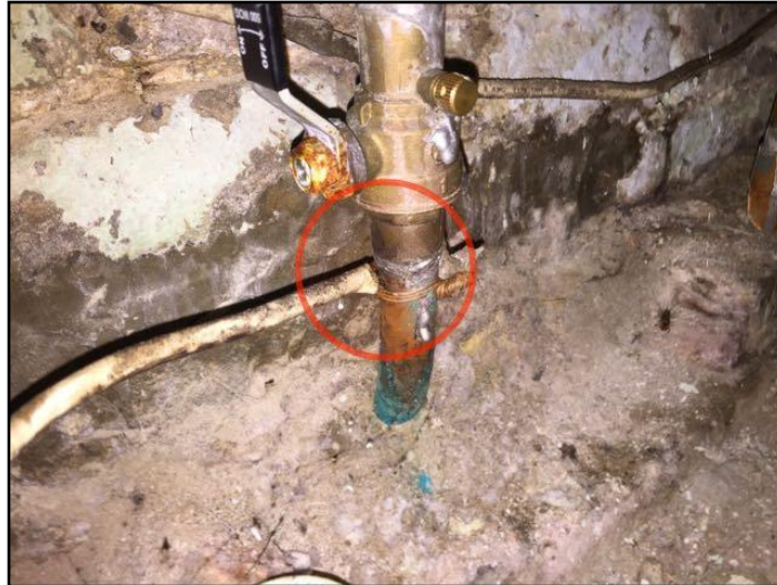
Poor connections/clamp missing
