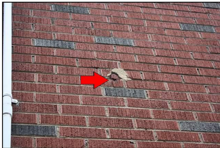
Gap at wall should be sealed
