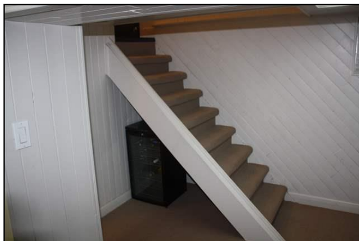
Railing - missing
