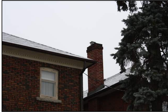
Masonry Cap - missing
