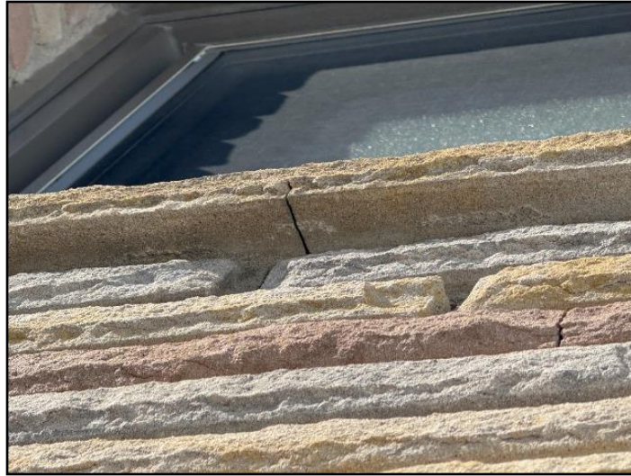
13. Patch sill cracks
