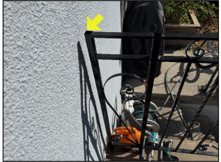
7. Not secured to wall
