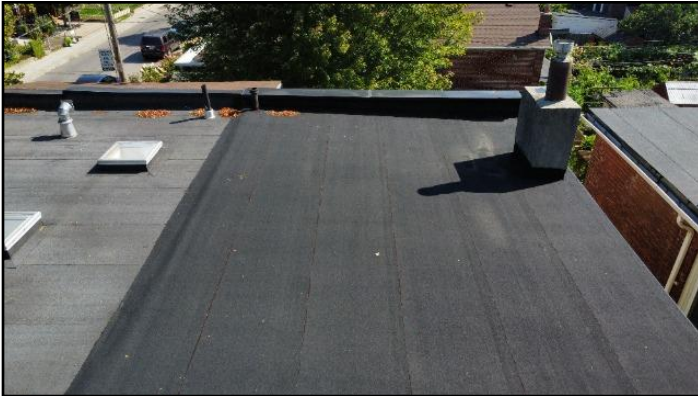
3. Modified bitumen membrane
