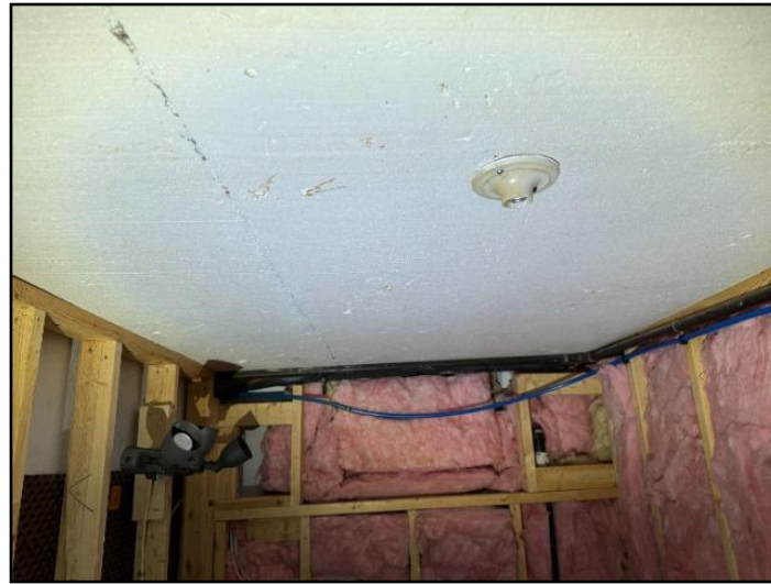
20. Combustible insulation exposed
