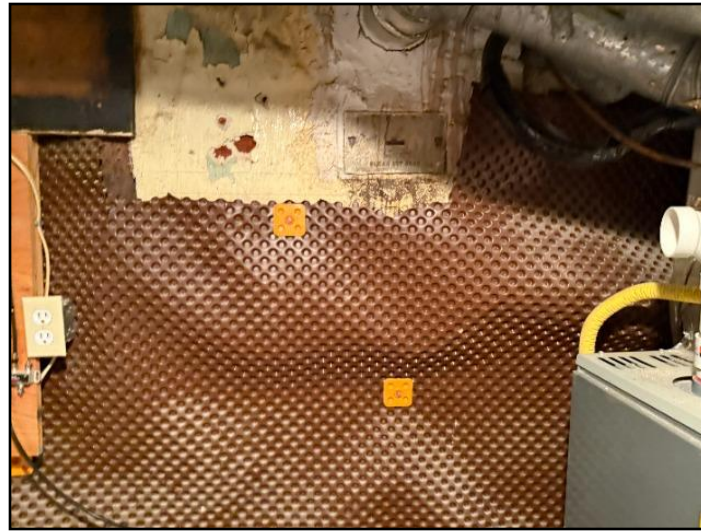
21. Interior dimple drainage membrane
