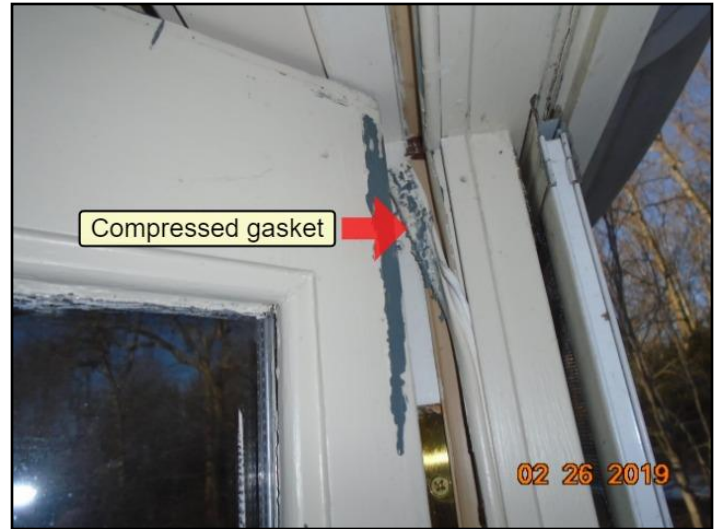
15. Air leaks/Back double door
