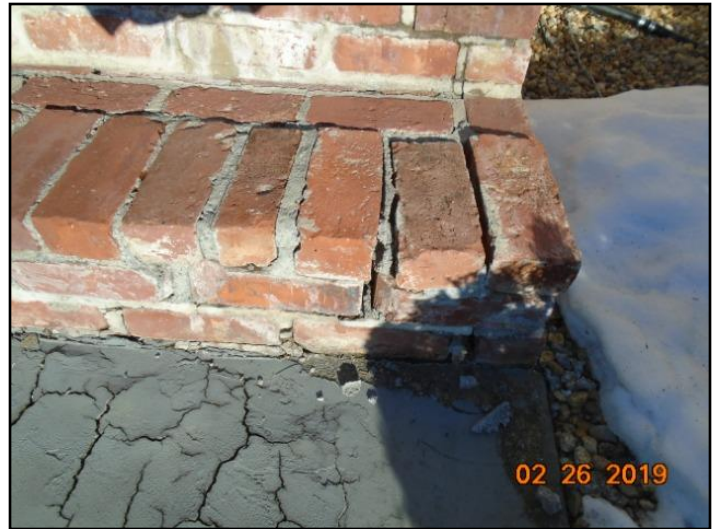
18. Repair loose bricks
