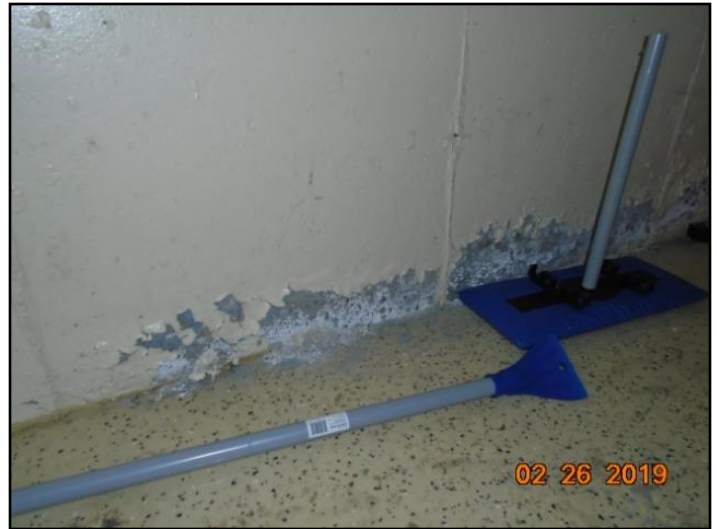
28. Salt damage to concrete
