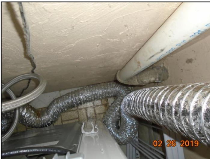
81. Dryer vent material not smooth wall
