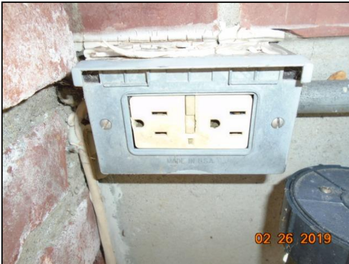
37. Missing cover/exterior
