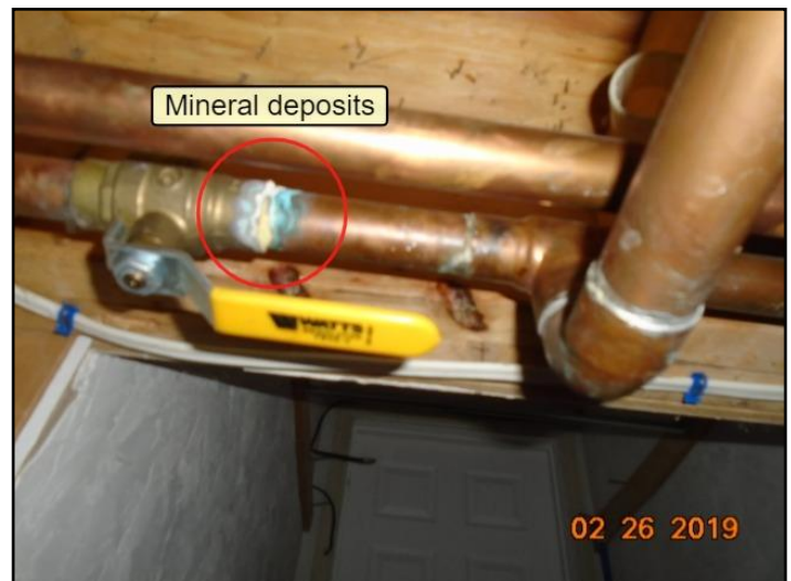
60. Corrosion/under stairs
