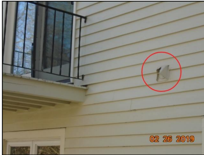
80. Damage/vent cover
