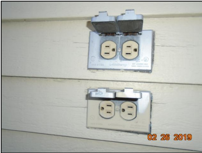
35. No GFCI location determined
