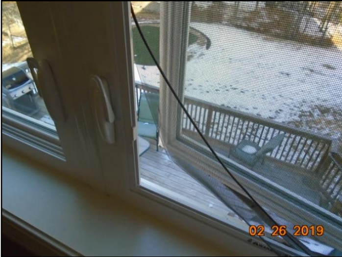
68. Left screen missing/right screen damaged
