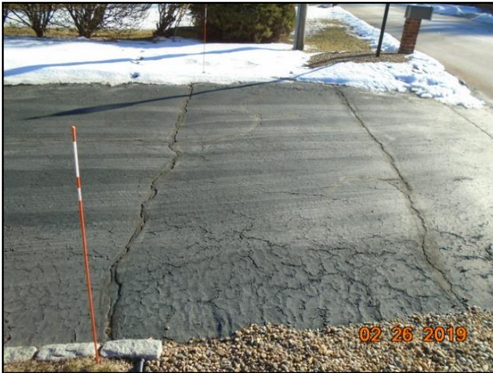
24. Seal driveway cracks and surface
