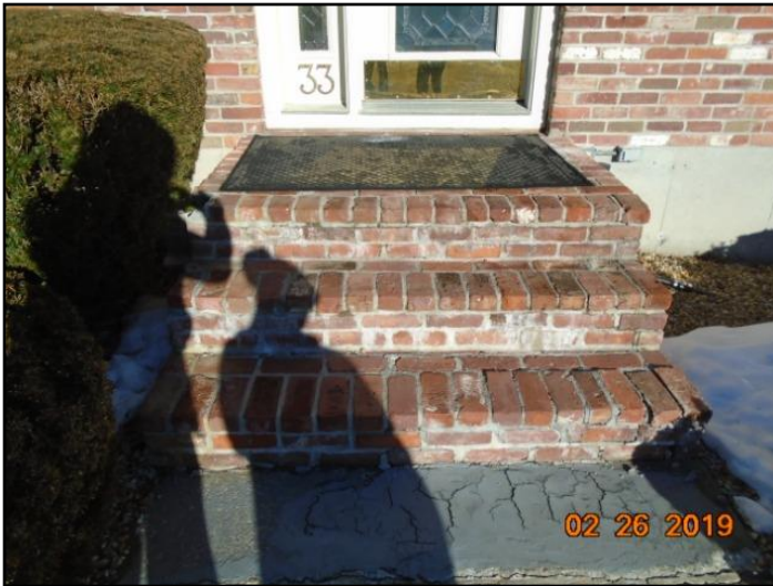
17. Repair loose bricks
