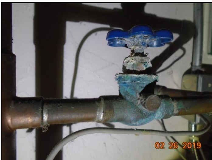
59. Corrosion/above boiler
