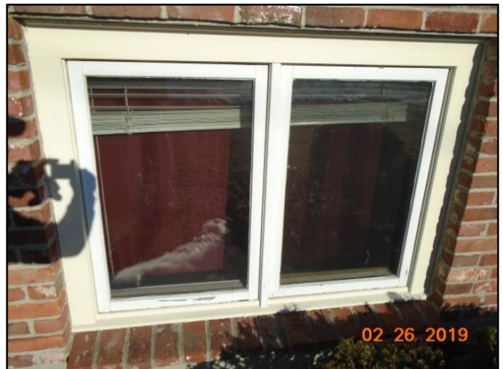
9. Paint and Caulking - deteriorated / missing
