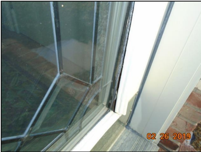
14. Air leaks/trim loose around glass
