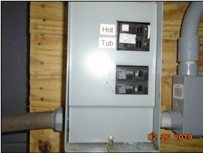
42. Breakers/Hot tub under deck
