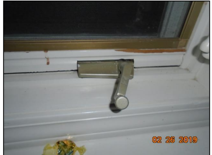
71. Inoperative/crank broke
