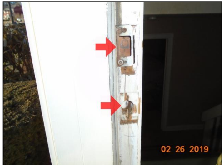
13. Repair/replace strike plates
