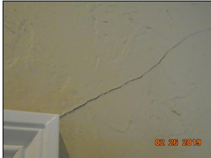
66. Small crack at doorway
