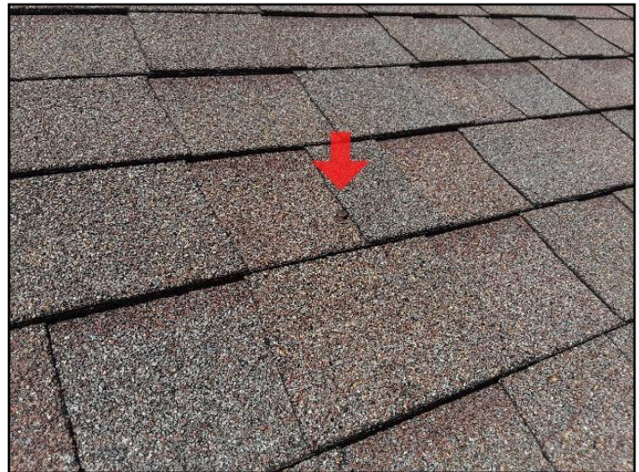
4. Exposed fasteners
