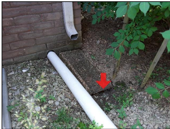
5. Wash-out beneath splash block
