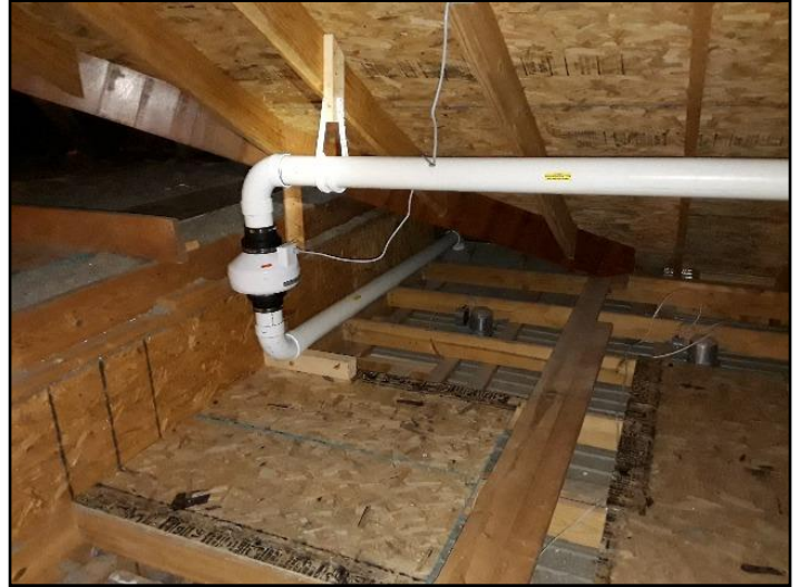
23. Radon in-line exhaust fan in the attic
