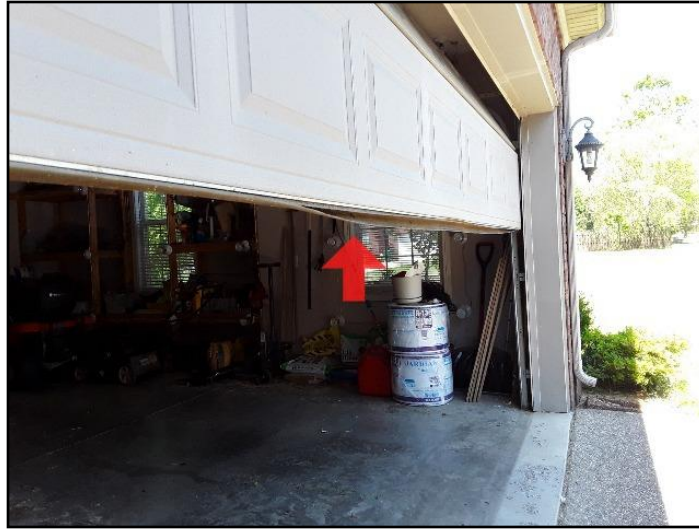
10. Damaged weather strip
