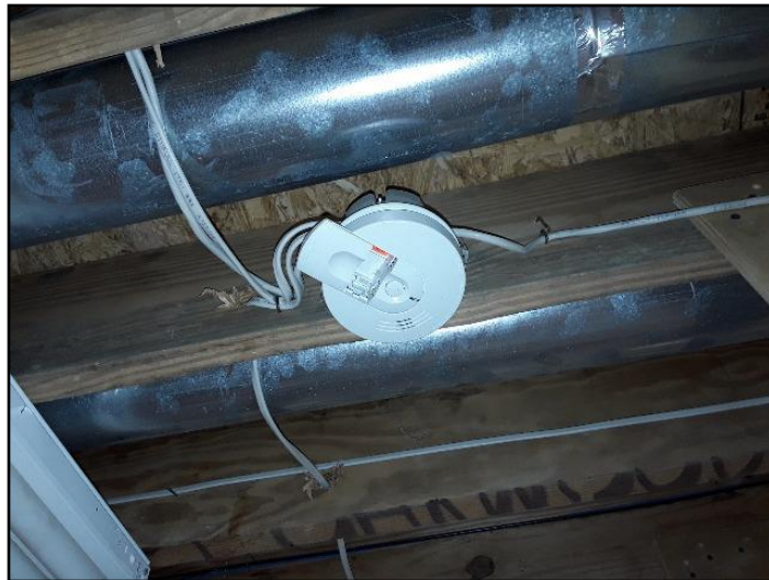
14. The backup battery has been removed
