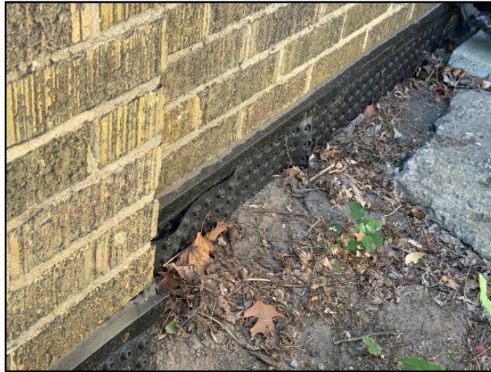
31. New dampproofing material
