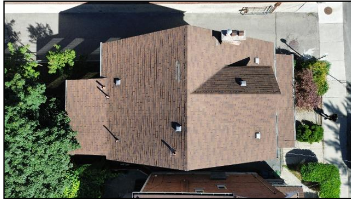
1. Asphalt shingles
