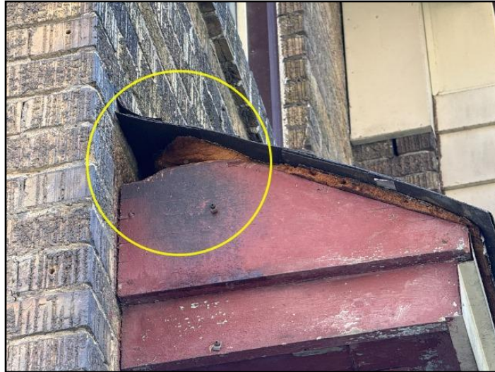
8. Flashings missing
