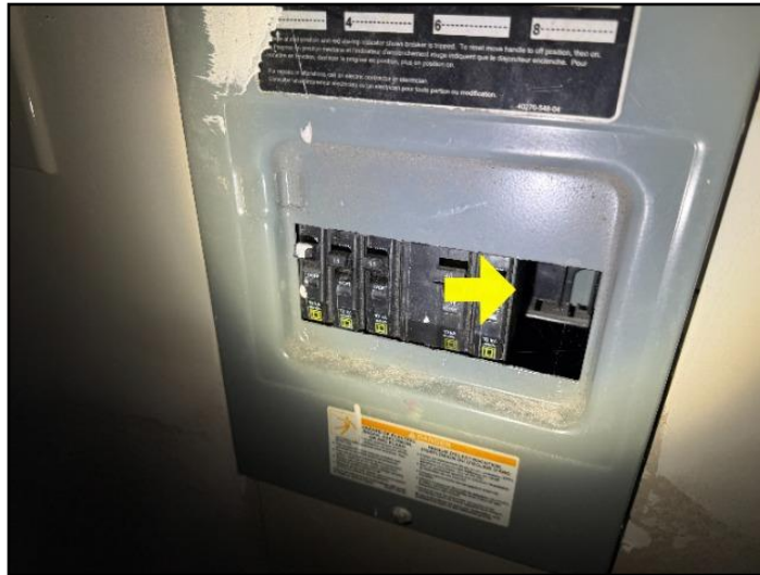
22. Unprotected Opening(s)
