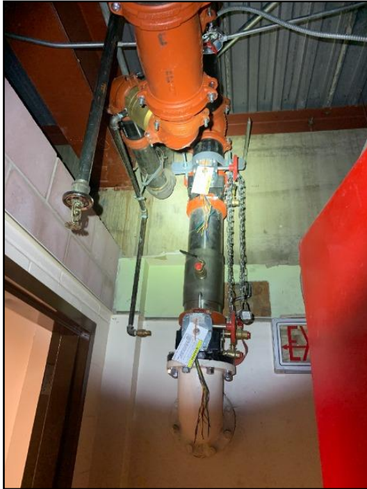
124. Example main fire protection sprinkler pipe
