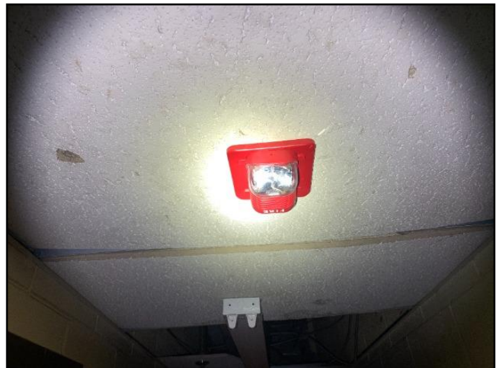
127. Example Fire Alarm Horn/strobe
