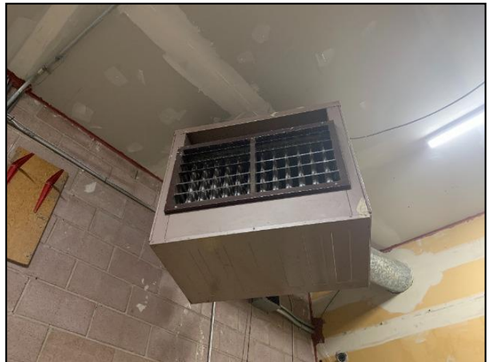
10. Example of unit heater #4 Shipping
