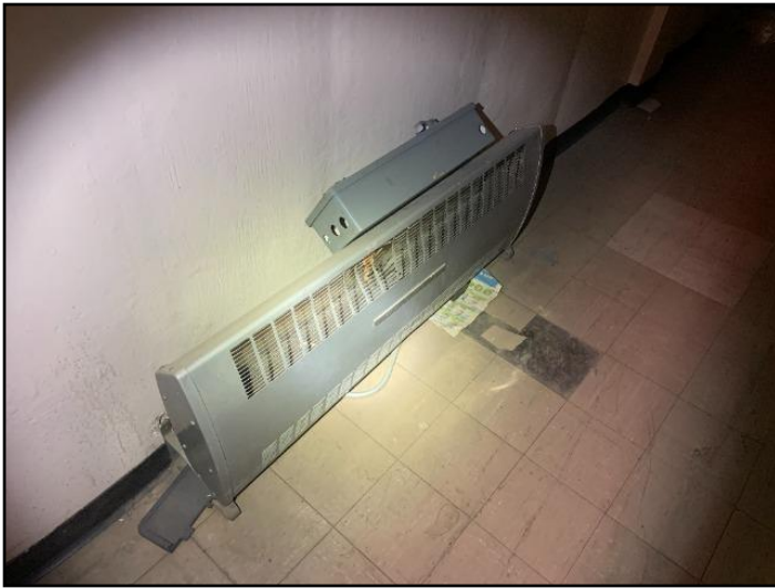
11. Example electric heat basement
