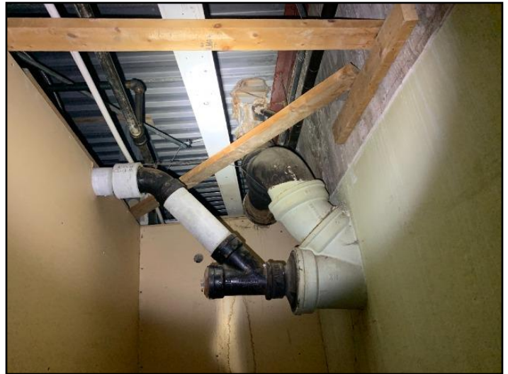
65. Example main waste piping
