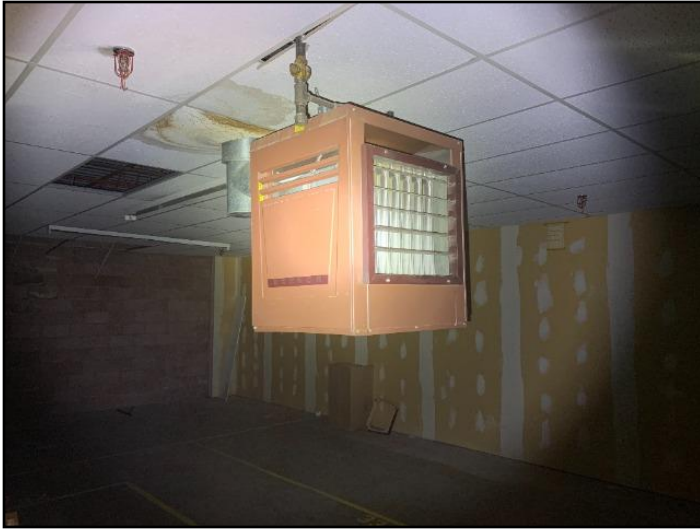
7. Example of unit heater #1 warehouse
