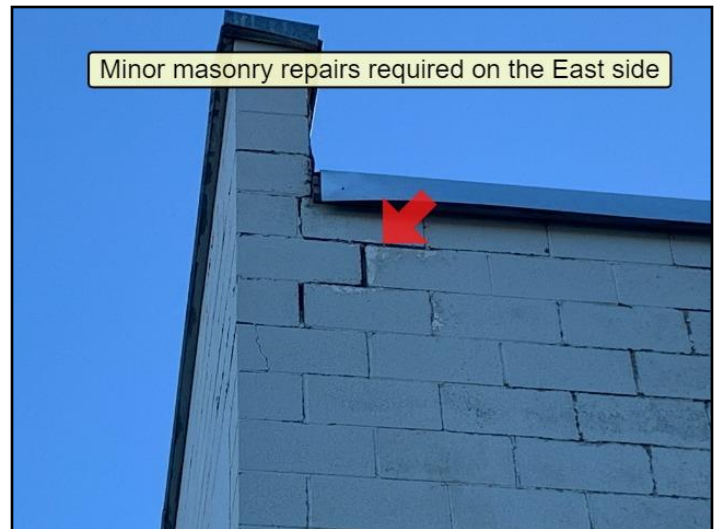
148. Typical settling cracks
