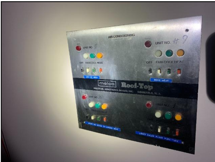
9. Example heating system controls
