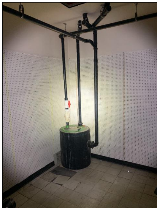
62. Example solid waste pump
