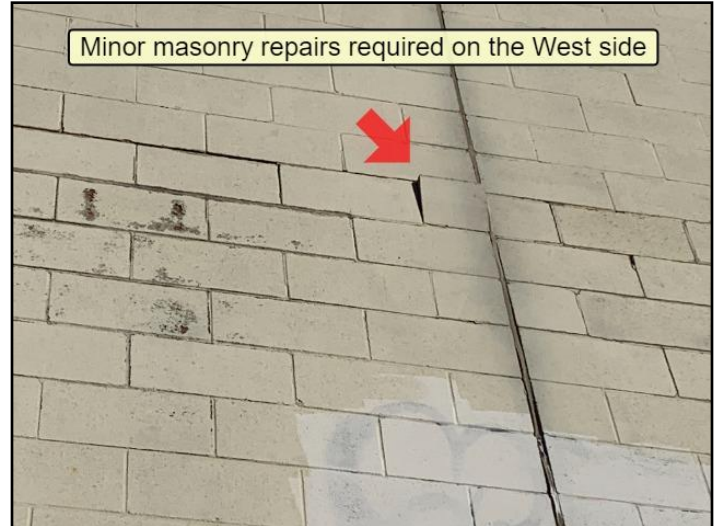
146. Typical settling cracks
