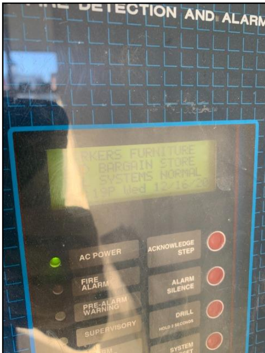
126. Example Fire Alarm Panel
