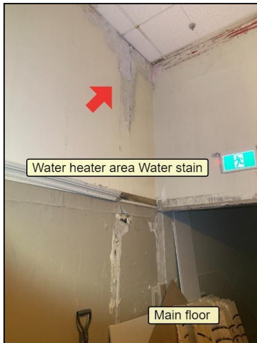
92. Water heater area Water stain
