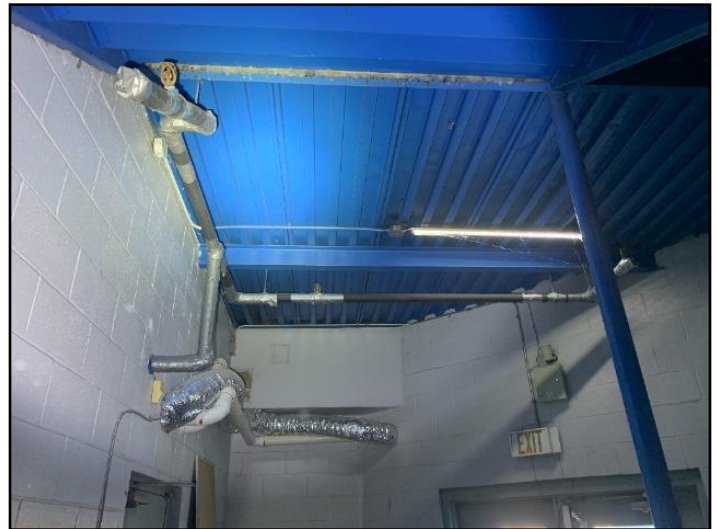
136. Example supported by steel beams and columns
