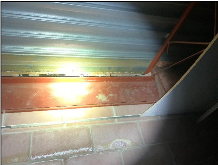
139. Example supported by exterior walls
