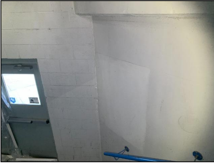
137. Example poured-concrete and cinder block
