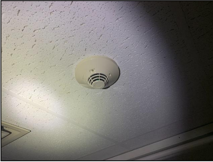
128. Example Fire Alarm smoke detector
