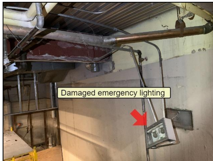
105. Damaged emergency lighting
