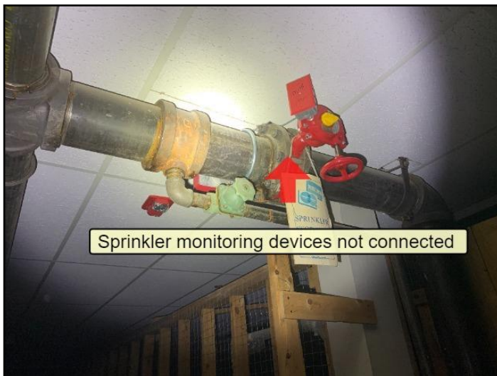
108. Sprinkler monitoring devices not connected
