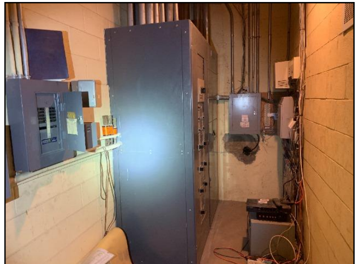
29. Example main electrical distribution
