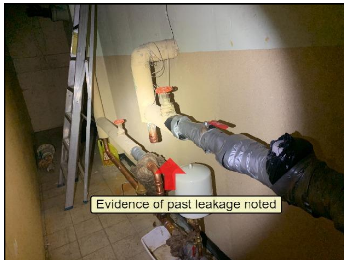
39. Evidence of past leakage noted
