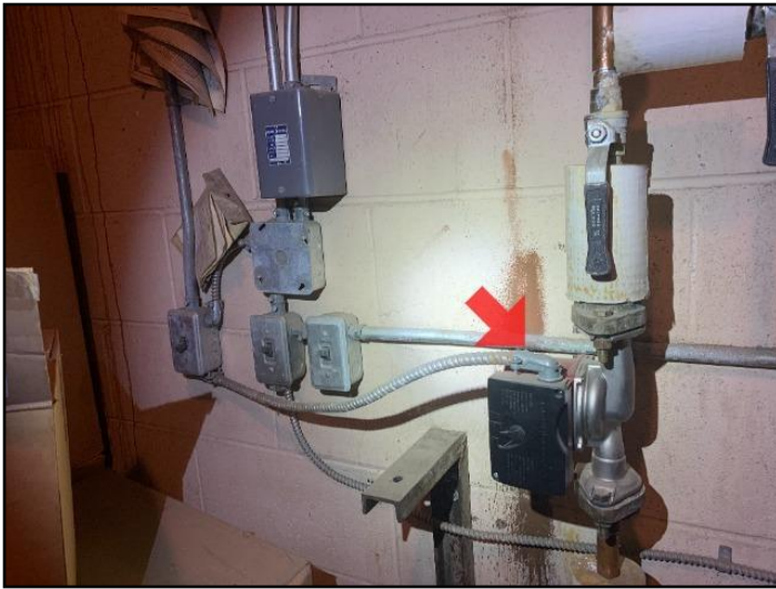
60. Example water pressure booster pump
