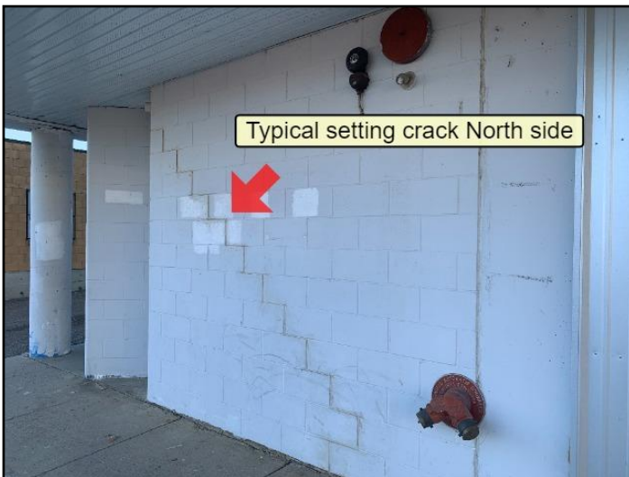
147. Typical settling cracks
