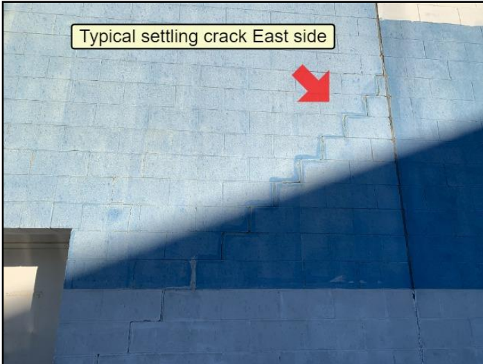
145. Typical settling cracks
