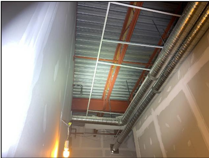
135. Example supported by open web steel joists
