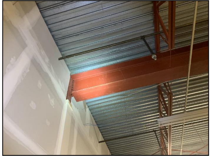
142. Example steel beams supporting steel deck
