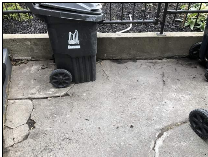
11. Improper slope or drainage
