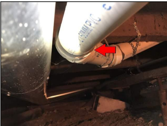
23. Poor connections, minor drip from exhaust
