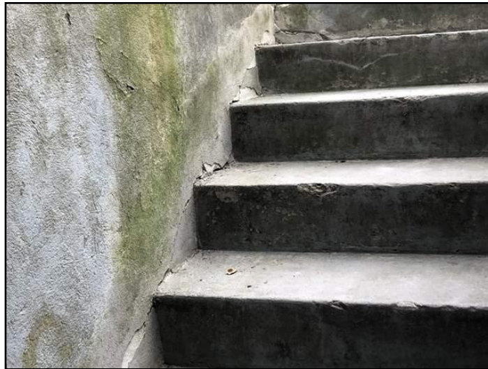
6. Parging damaged or missing
