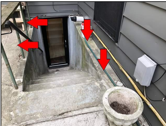
8. Guard and handrail problems
