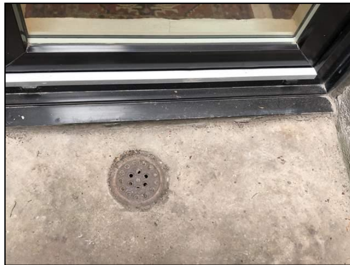
10. Door threshold missing, too low, not...
