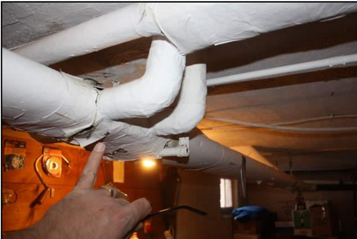
19. The insulation on the boiler or heating...
