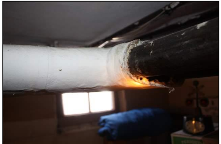
20. The insulation on the boiler or heating...
