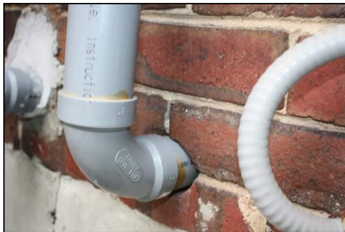
6. Caulking missing or ineffective
