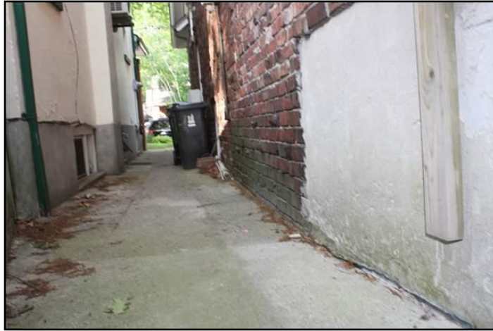
16. Improper slope or drainage
