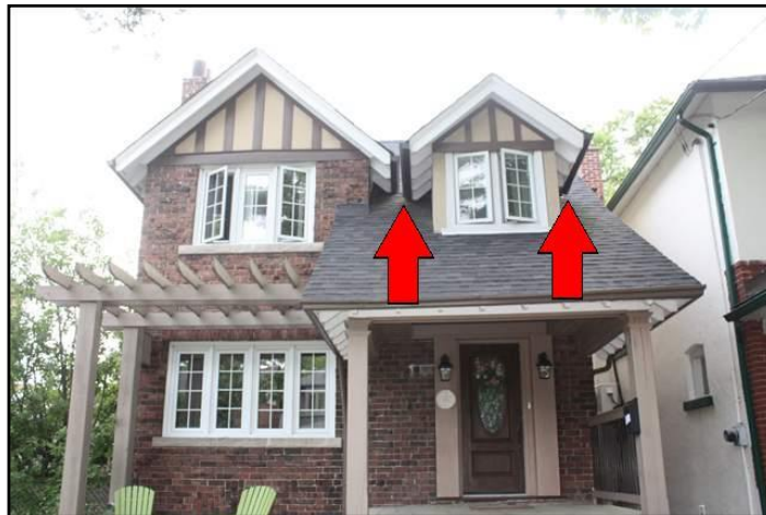
3. Discharge onto roofs
